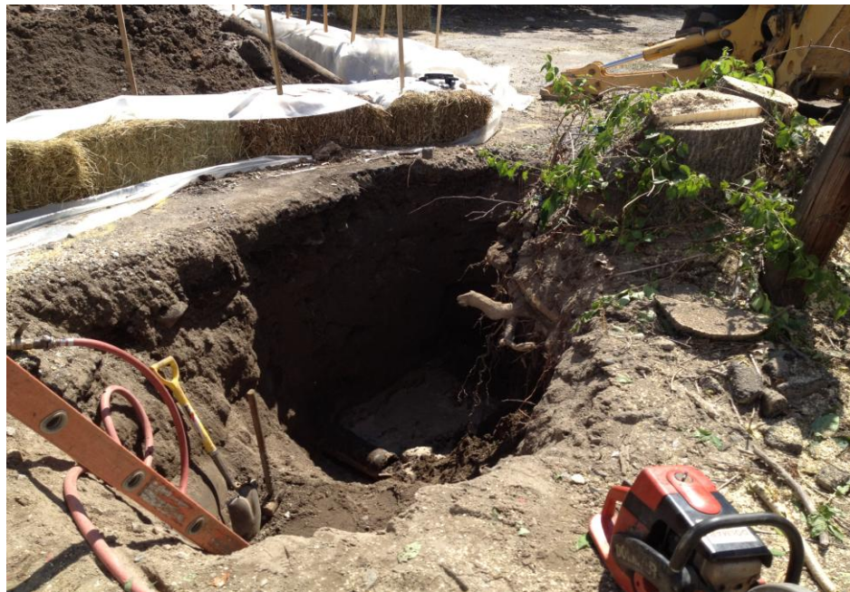
Excavation and stockpiled material prior to hydrant install. June 26, 2012.
