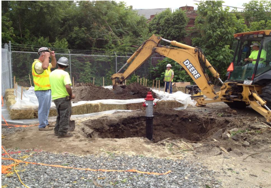
Excavation with hydrant installed. Excavation is being backfilled. June 26, 2012.
