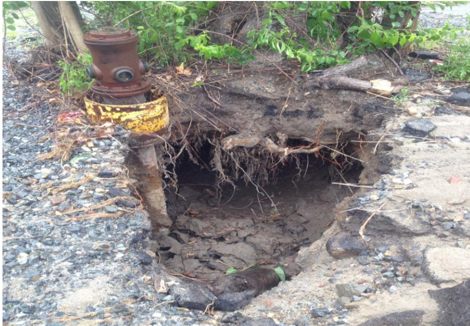
Hydrant and Valve Block prior to replacement/repair. June 4, 2012.
