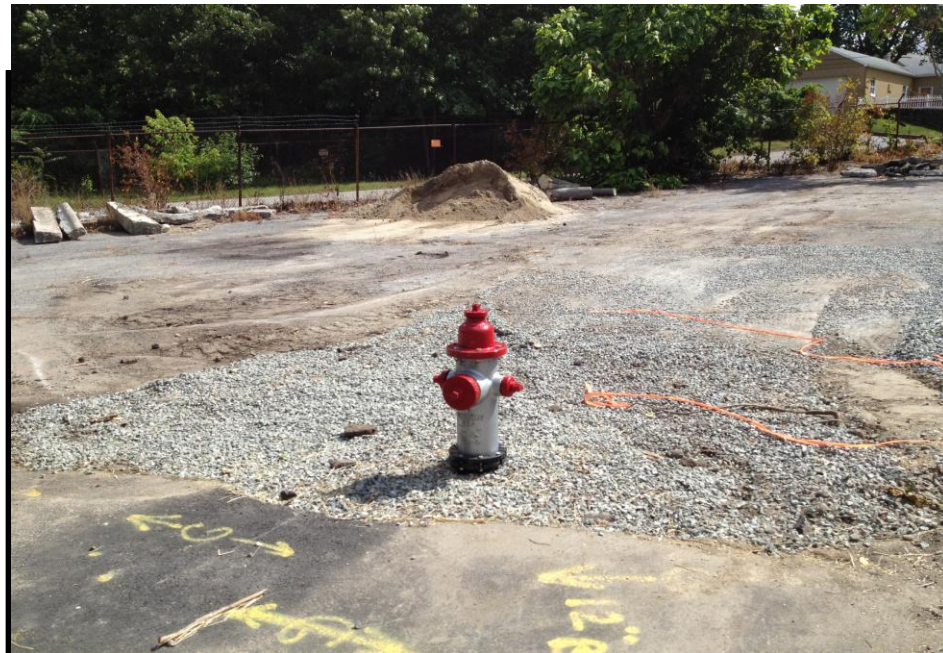
Final new hydrant and backfilled area. June 26, 2012.
