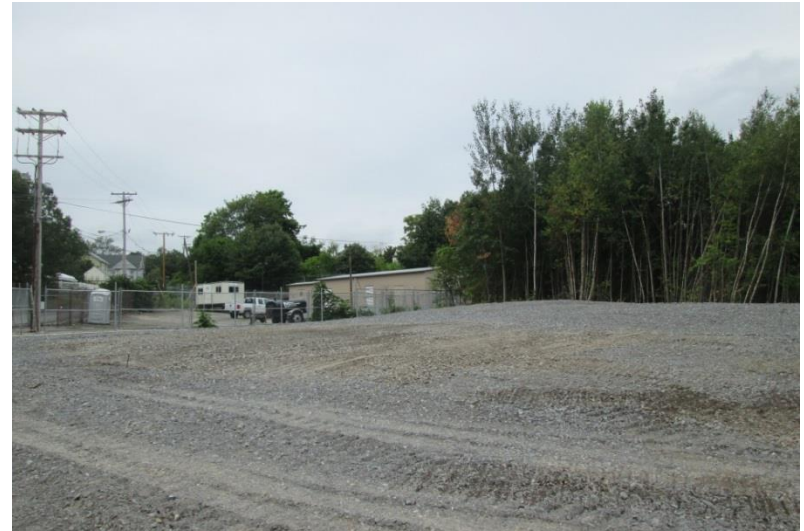
PHOTOGRAPH 8 – Final grading looking west
