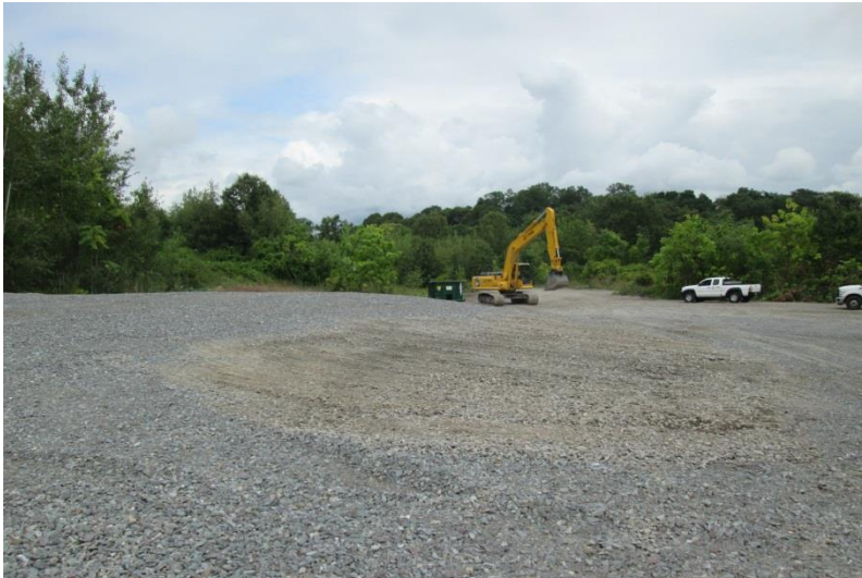
PHOTOGRAPH 7 – Final grading looking east
