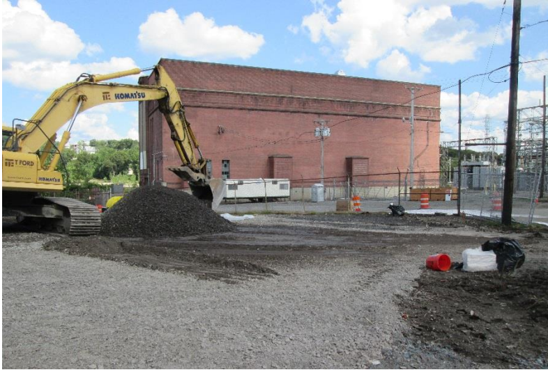
PHOTOGRAPH 5 – Looking southeast, Beginning hydraulic fluid impacted soil excavation activities
