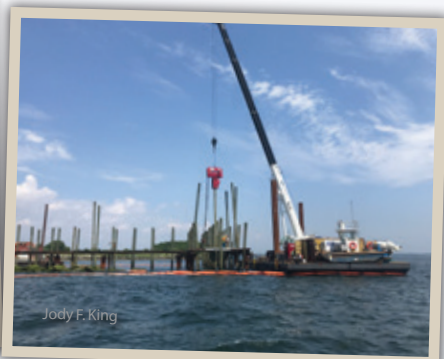
New timber piles being installed
