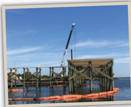
Pile bracing, part of pier decking installed
