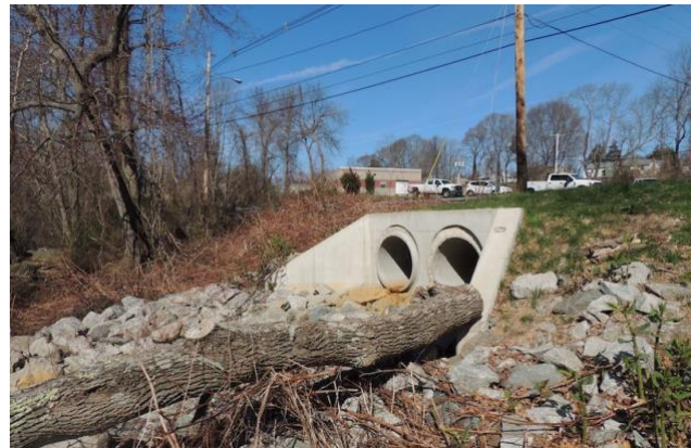
Culverts along bank of river near site of DV-01
