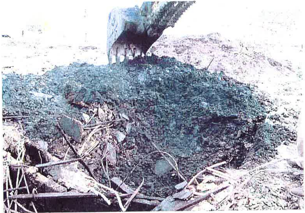
Stabilization of contents of Structure 19 using "speedi-dry".
