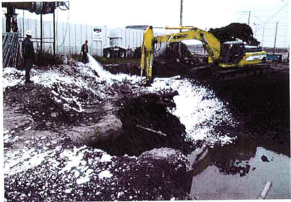
Area 2 excavation with CHES applying odor-suppressing foam.
