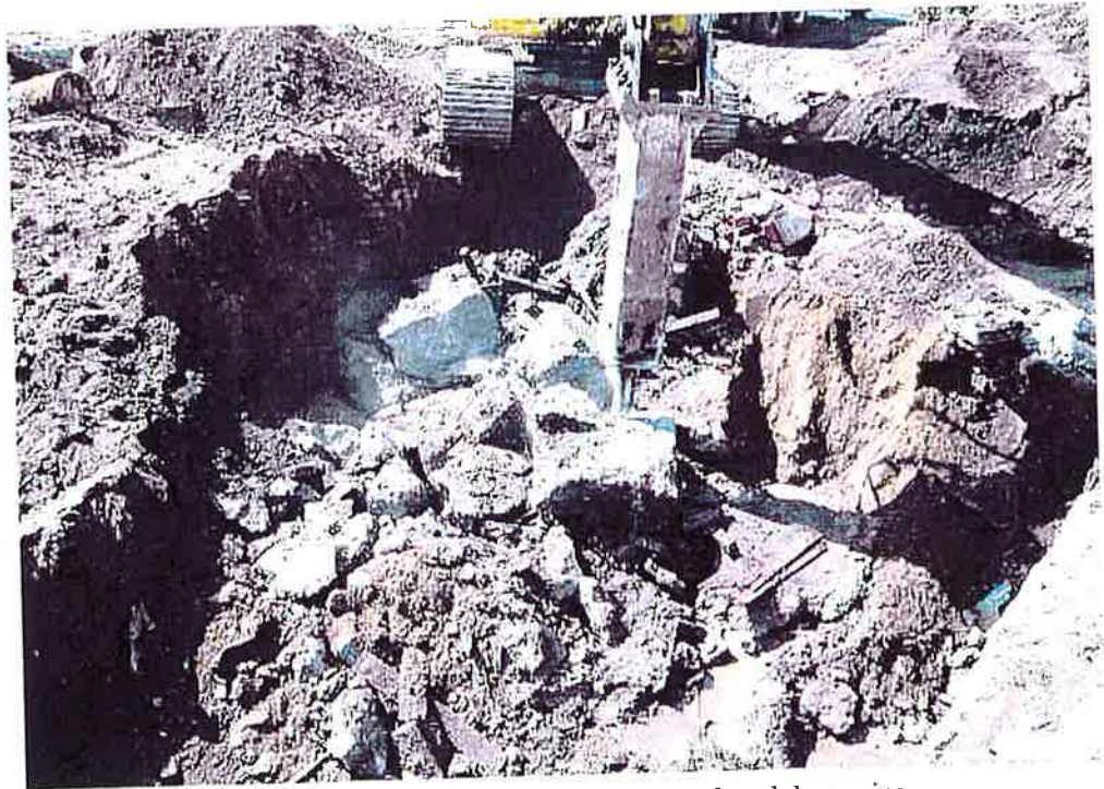
Demolition of subsurface structures next to knockdown pipe.
