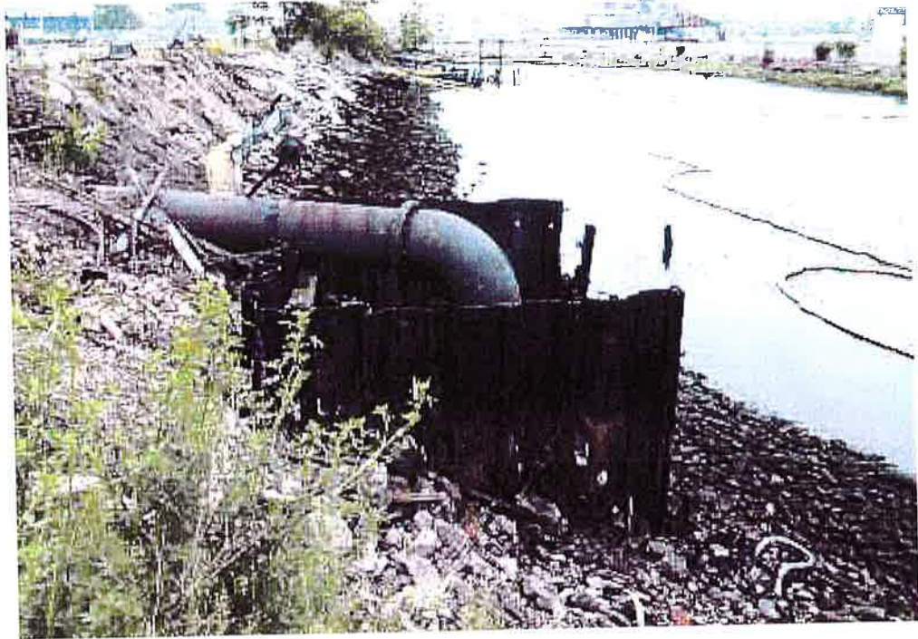
Salt-water intake structure before removal.
