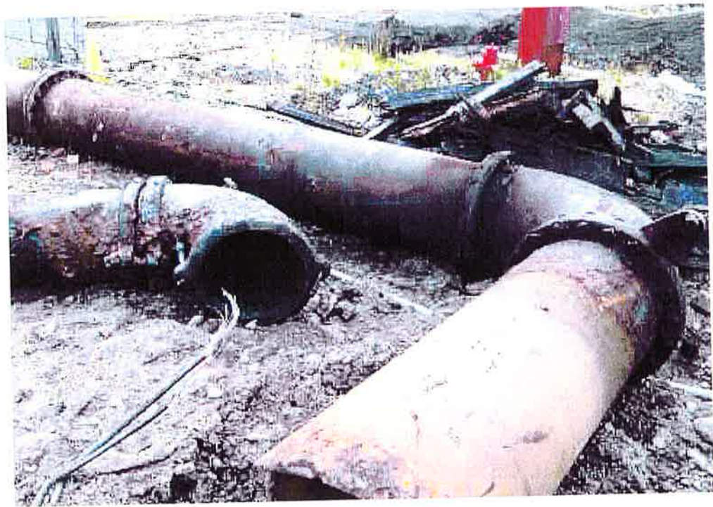
Salt-water intake structure piping after removal.
