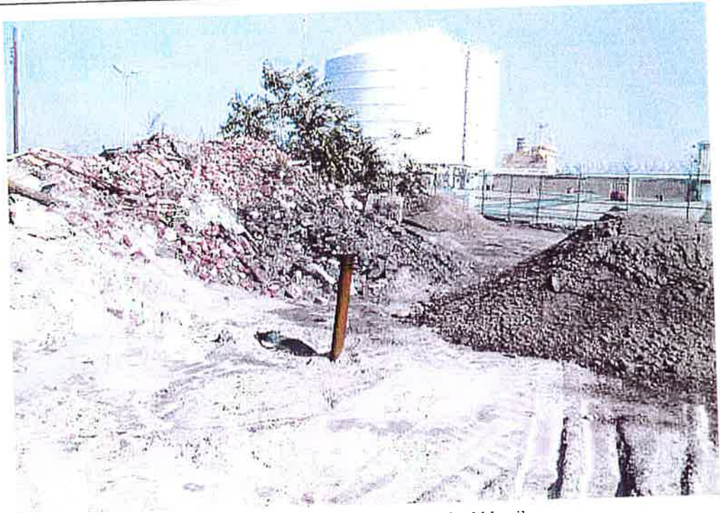
Partially demolished Building 9 and rubble piles.
