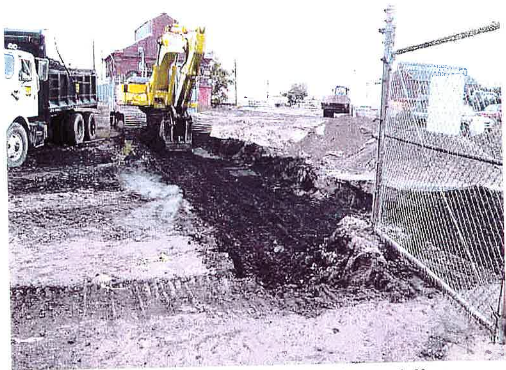
Additional surficial excavations outside area 3 following removal of fence.
