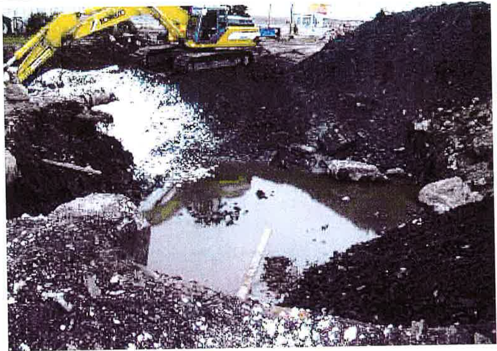
View of Area 2 excavation from west side.
