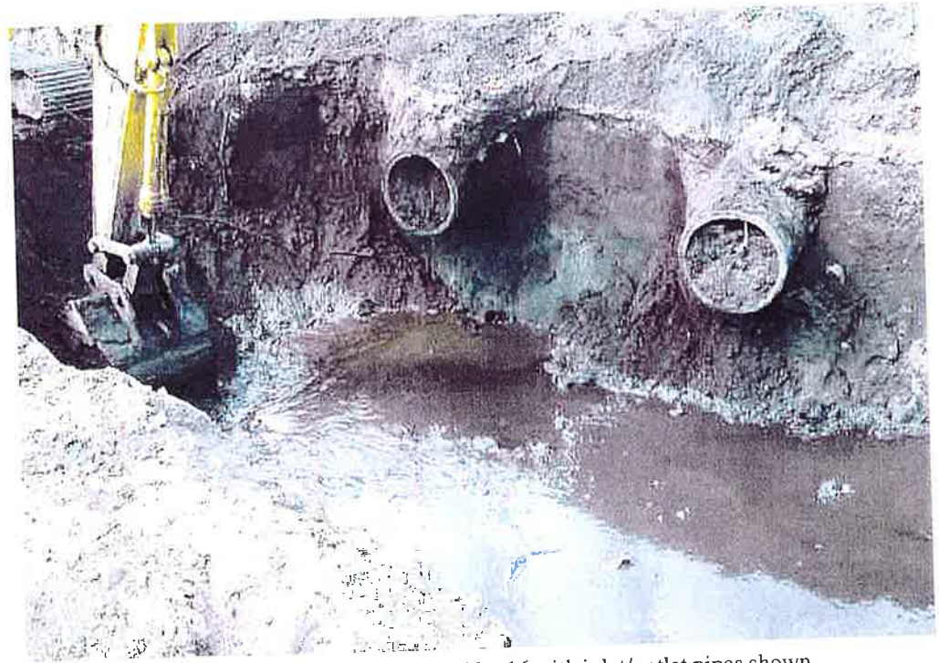
Excavation next to base of Gasholder 16 with inlet/outlet pipes shown.
