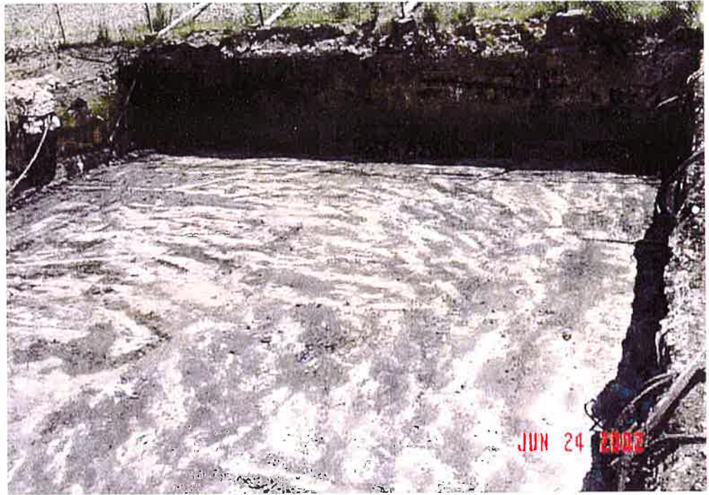
Western cell of Structure 3B after excavation/cleaning.
