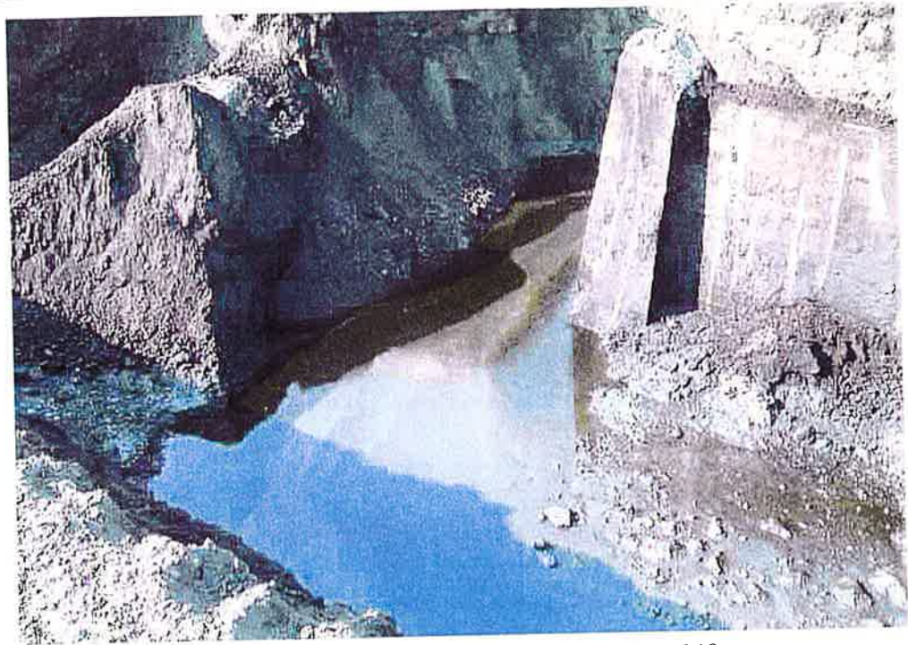
Subsurface soil excavation east of Structures 17 and 18.
