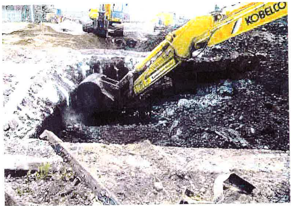
Excavation and stabilization of contents of Structure 18.
