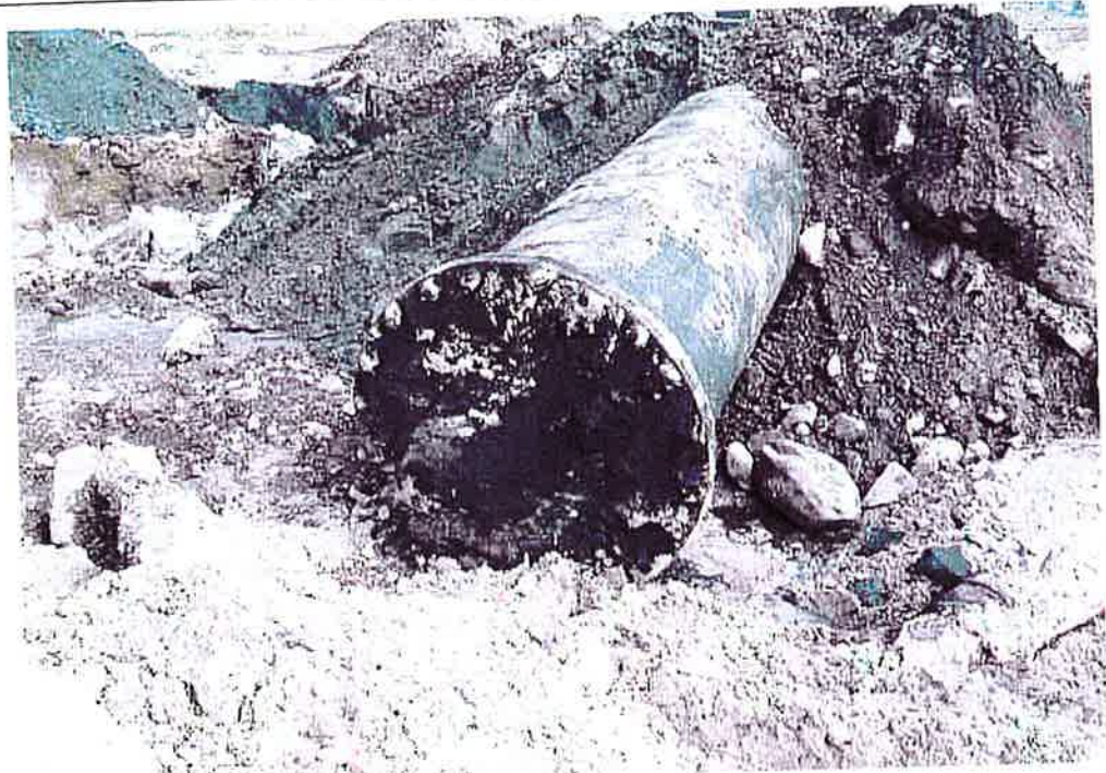
View of knockdown pipe after removed. (Note flanged bottom and rivets).
