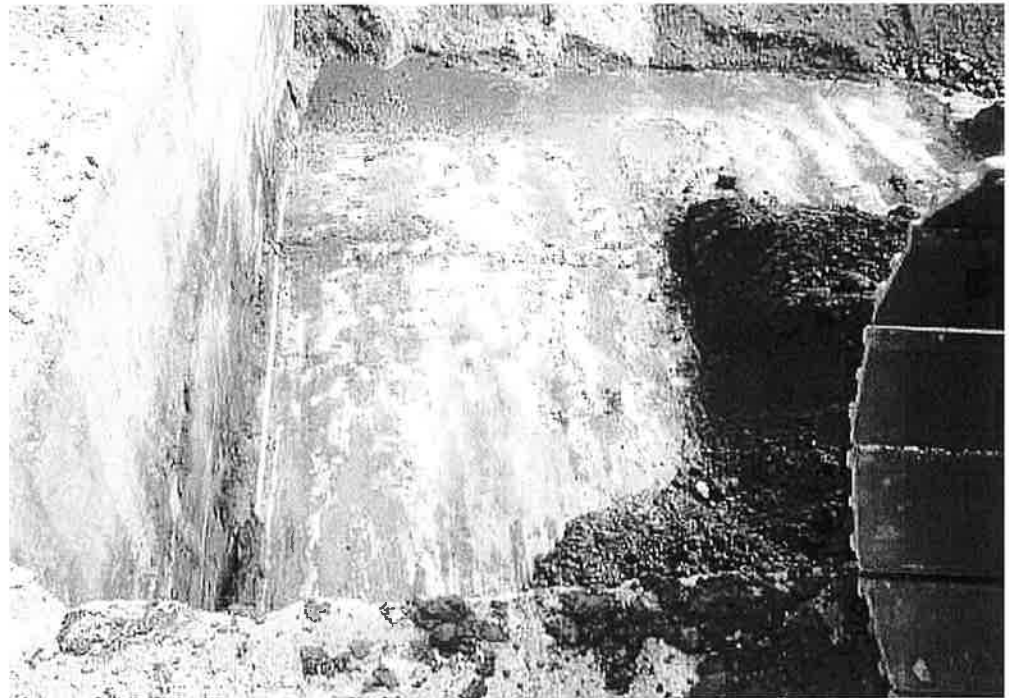
View of portion of bottom of Structure 17.
