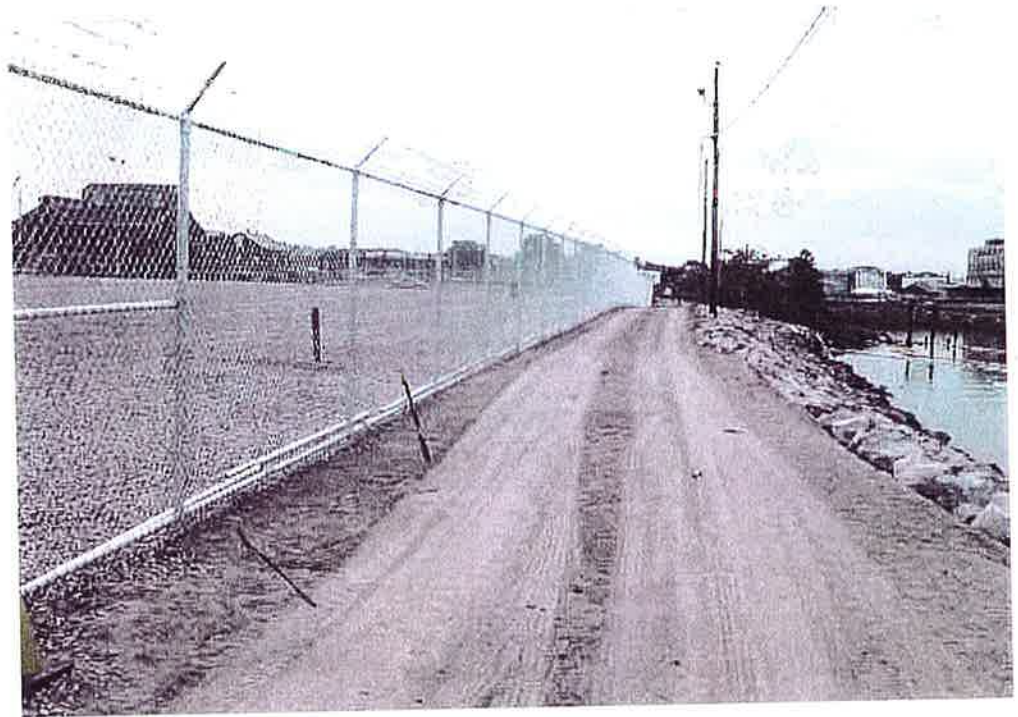
View of Access Road restoration.
