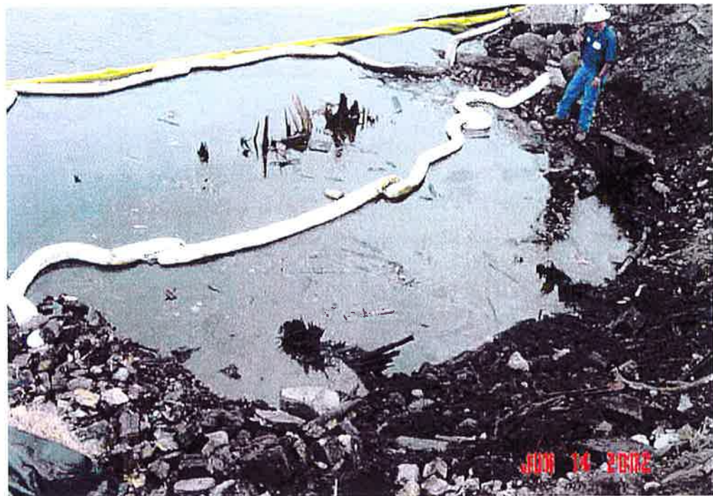
LNAPL recovery following removal of saltwater intake structure.
