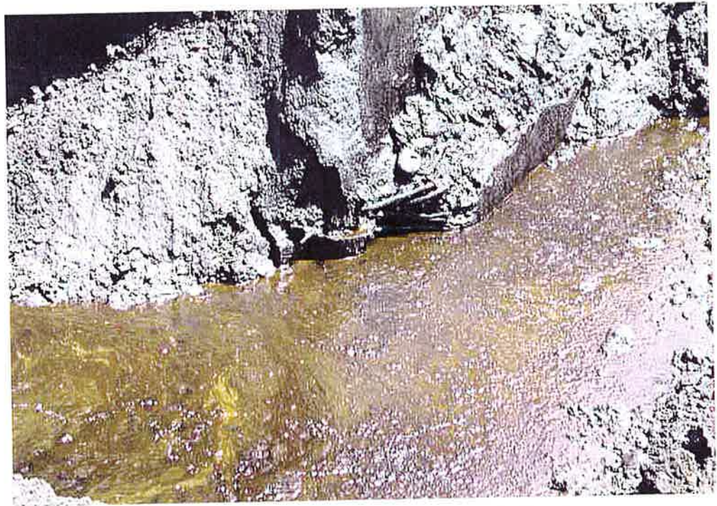
Accumulated groundwater and SPP at west end of trench.
