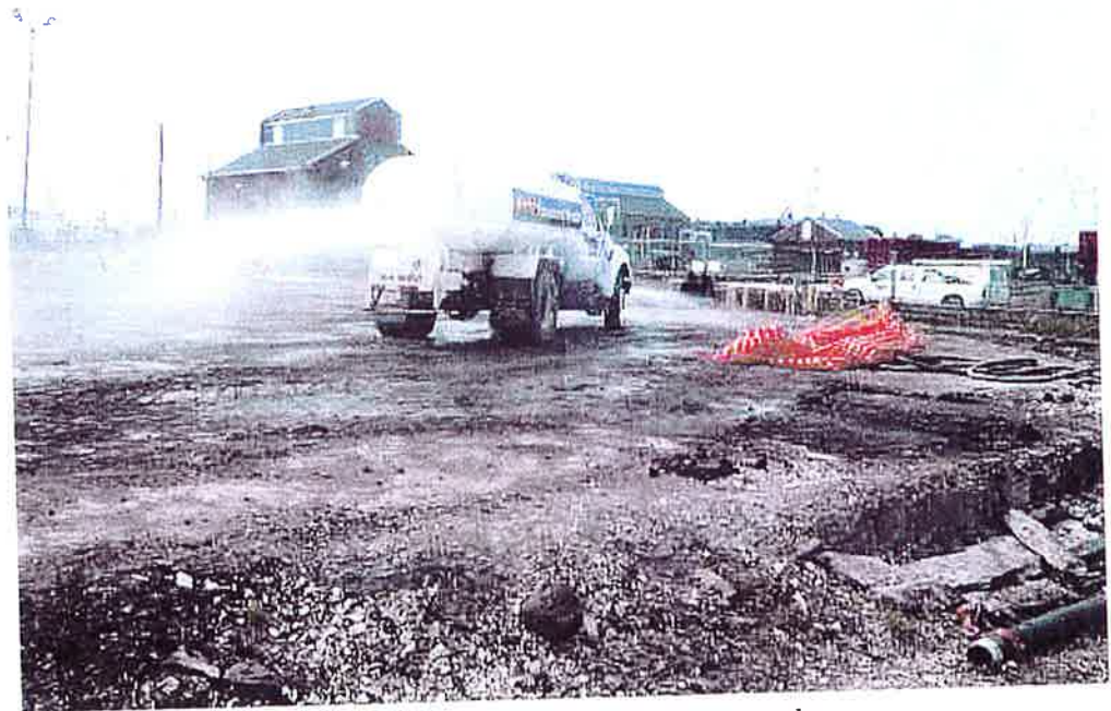
On Site dust suppression using water truck.
