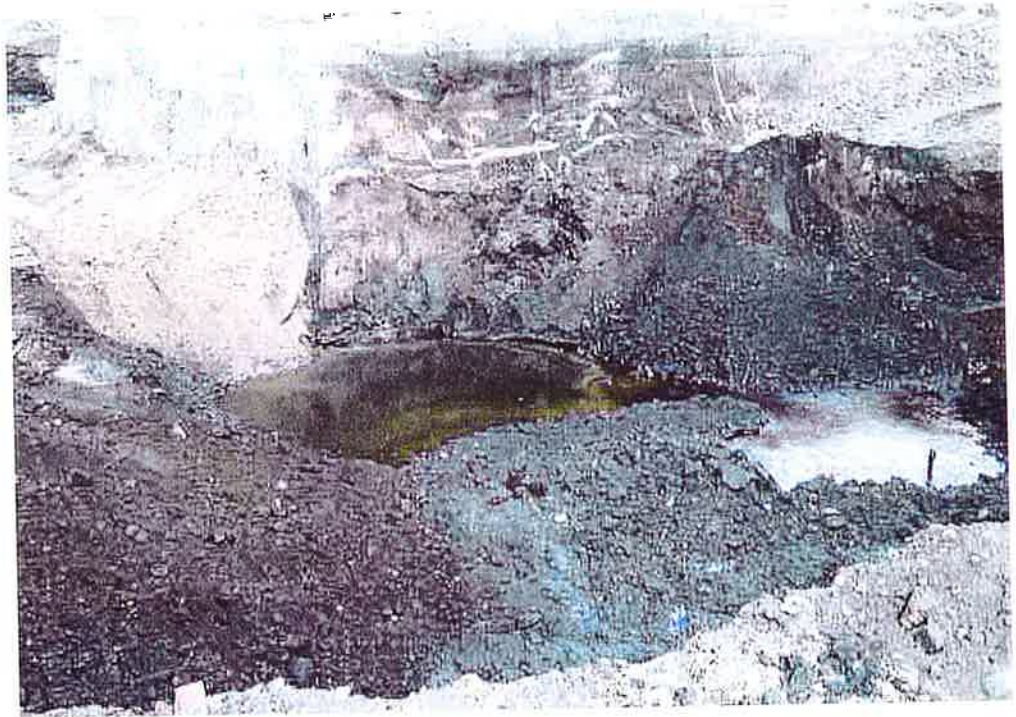
Clay backfill placed in front of Structure 17.
