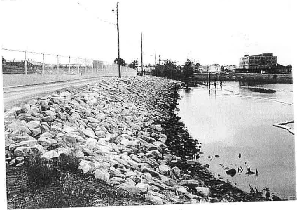
View of rip-rap restoration.
