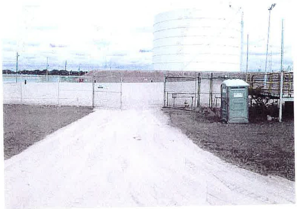
View of Area 3 restoration.
