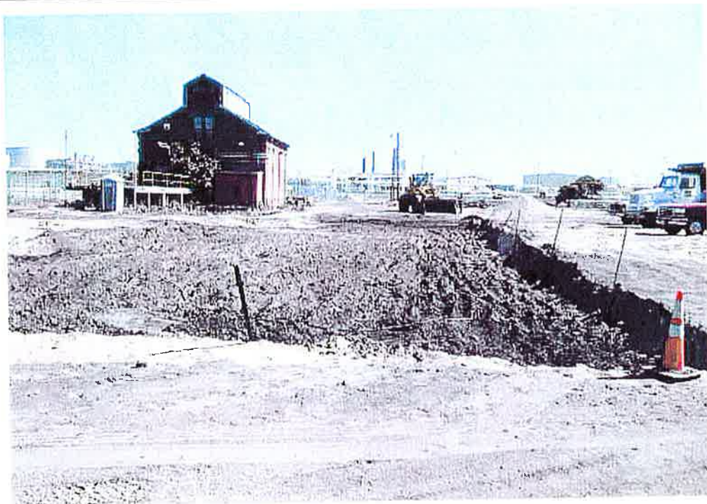
View of surficial excavation outside Area 3 and north of Building No. 20.
