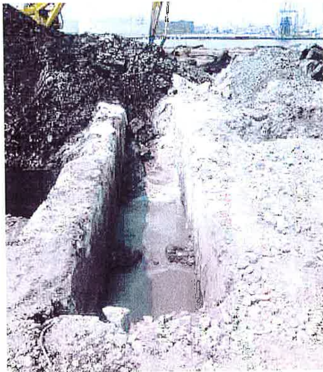
View of gap in Structure 18 separating eastern and western cells.
