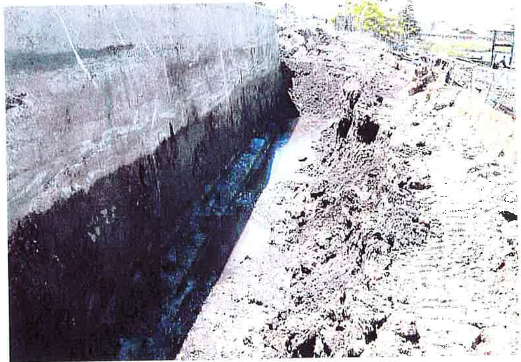
Seep trench excavated in front of Structure 17.
