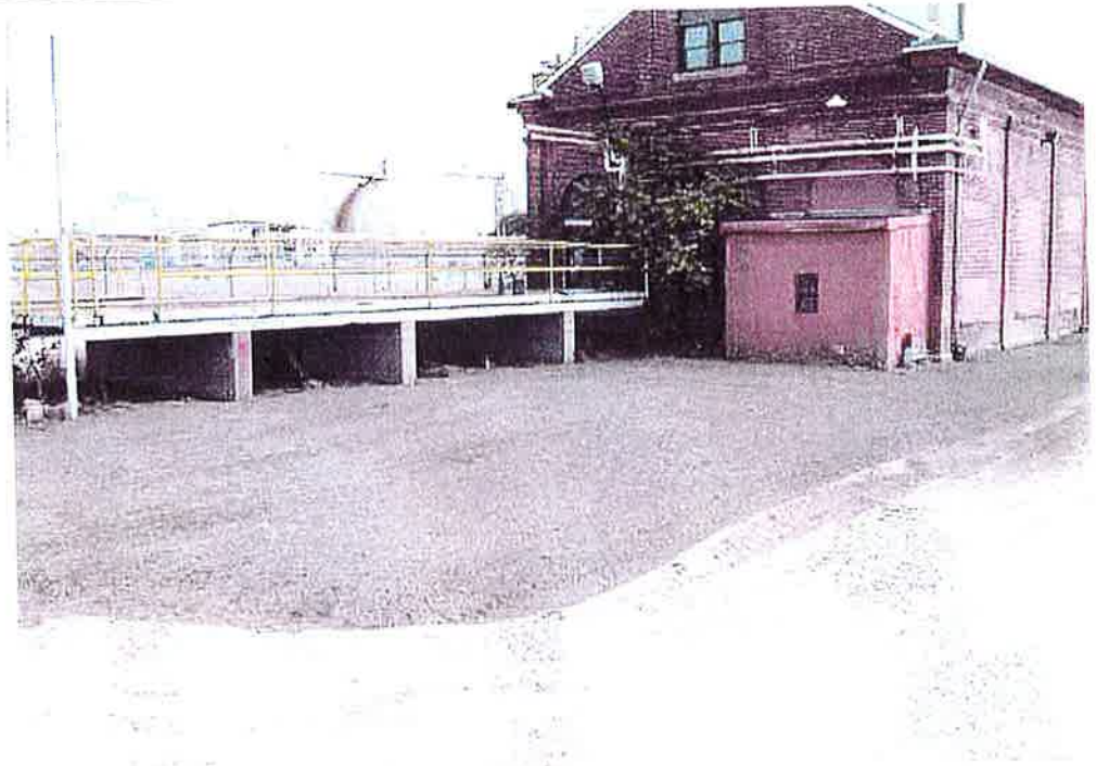
View of restored areas north of Building No. 20.
