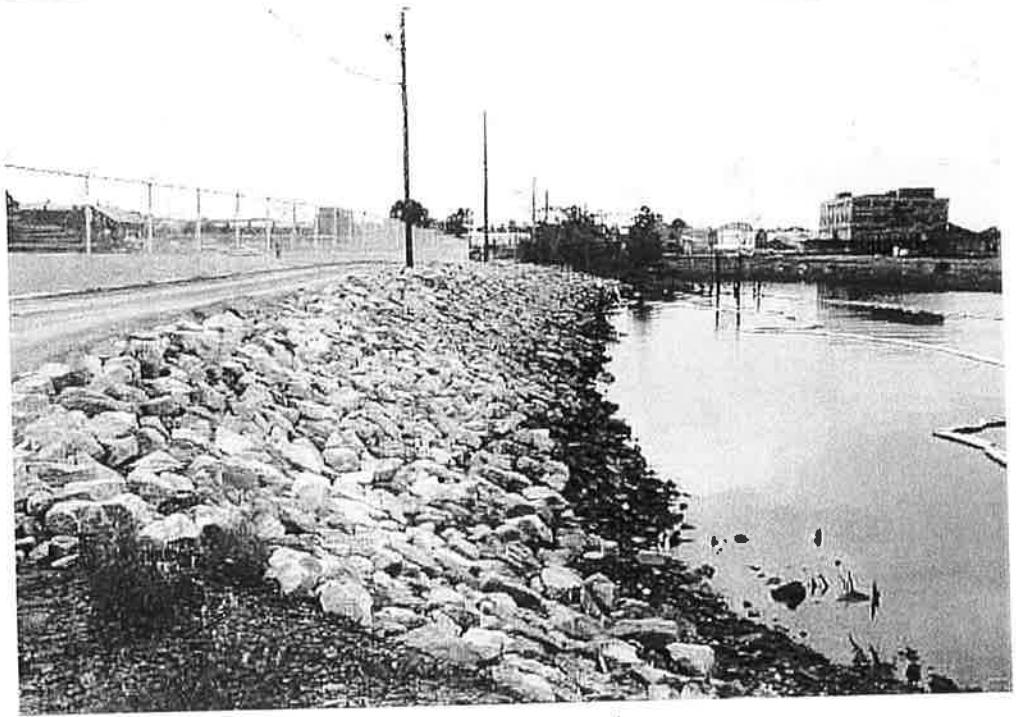
View of rip-rap restoration.
