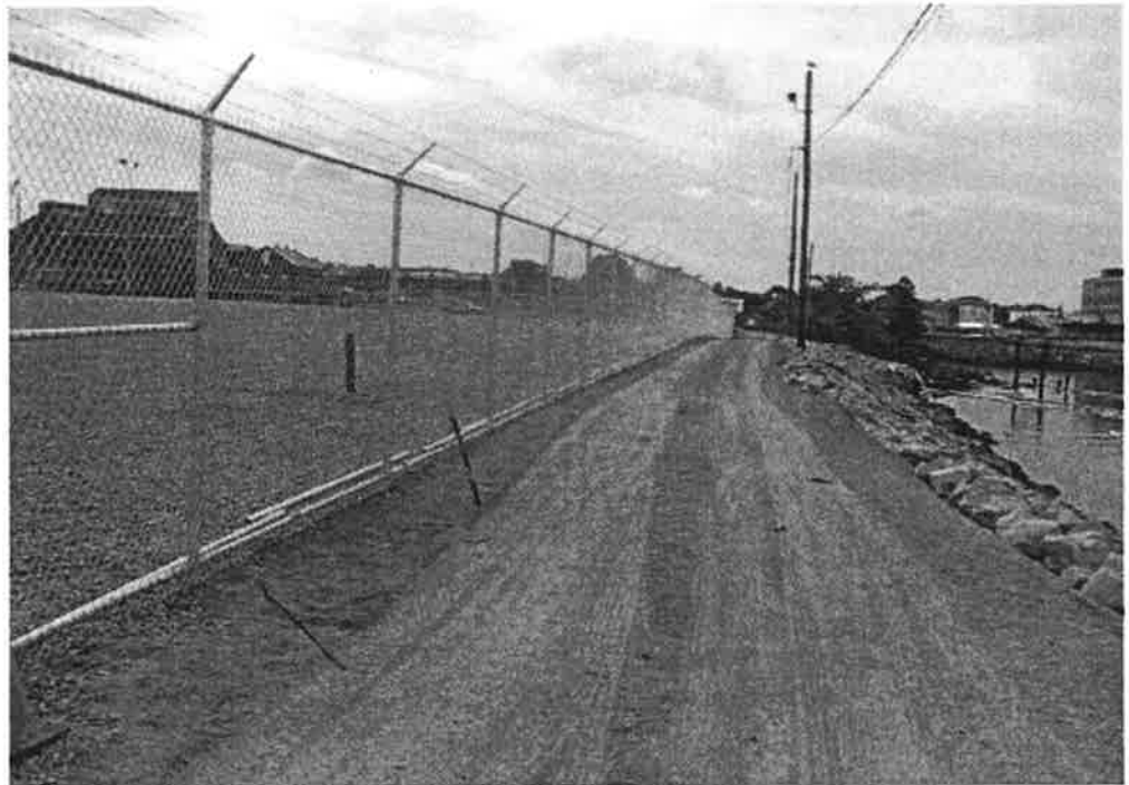
View of Access Road restoration.
