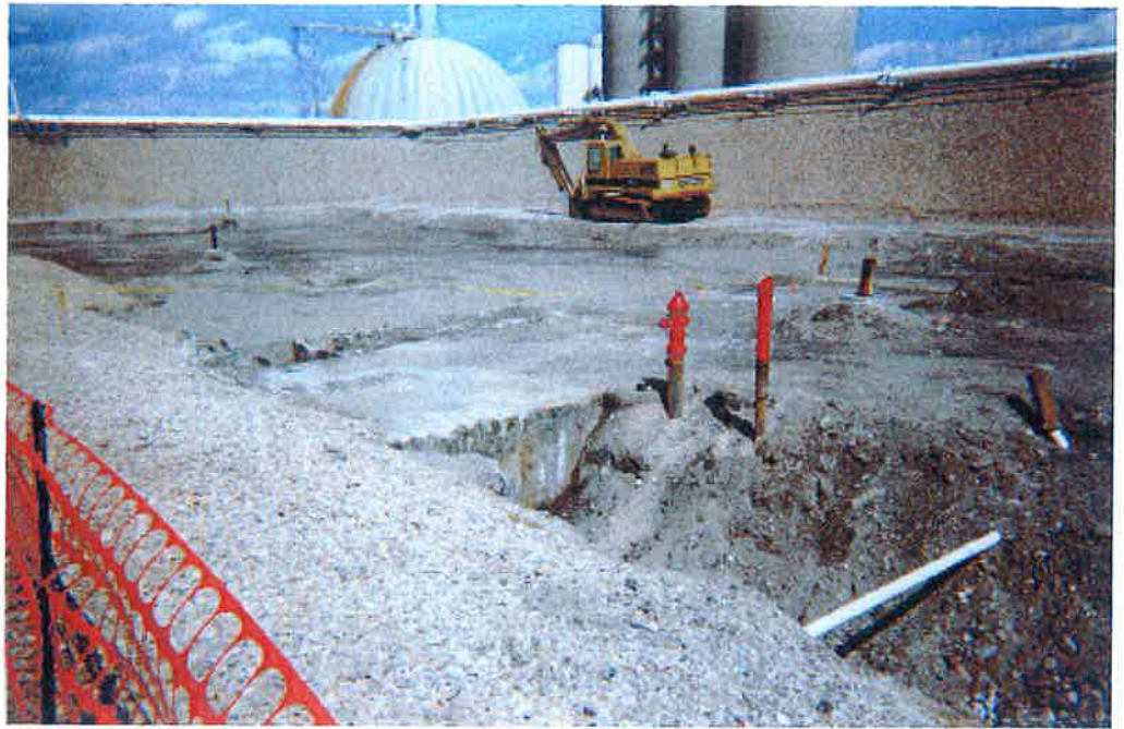
View of concrete pad looking southeast.
