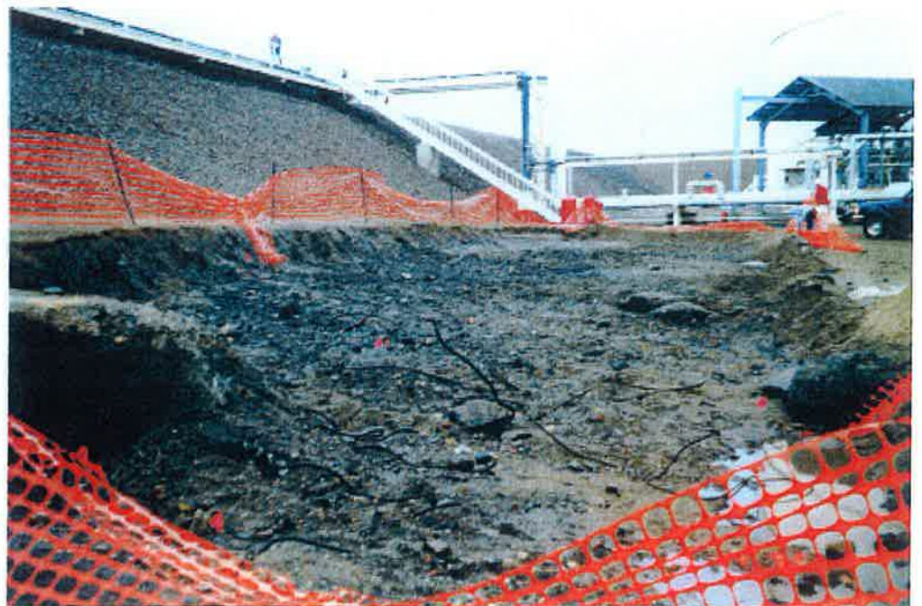
Surficial excavation in SALNG Area within the dike.
