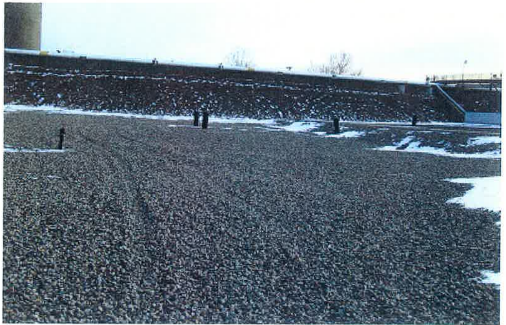
View of recent conditions of SALNG area looking to the south.
