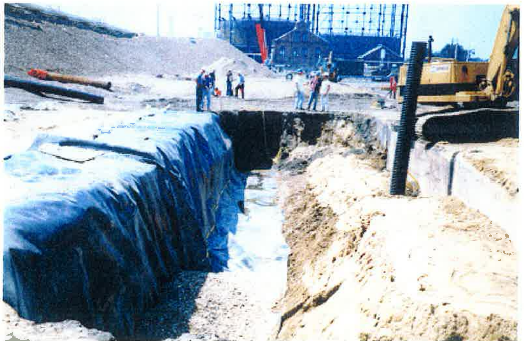
Backfill operations in SALNG Area looking westerly.
