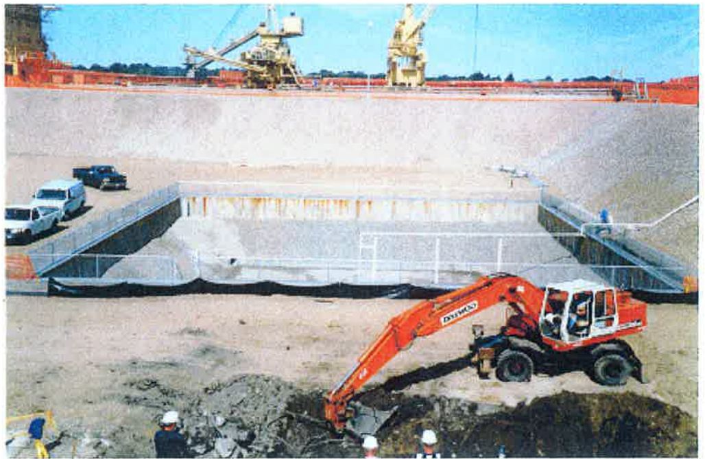
View of excavations in SALNG Area within the dike.
