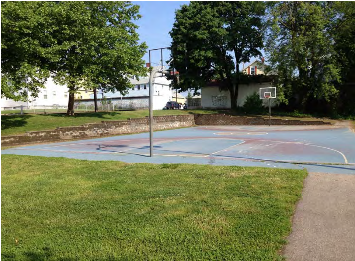
Retaining wall along western edge of the property at Chase Street
