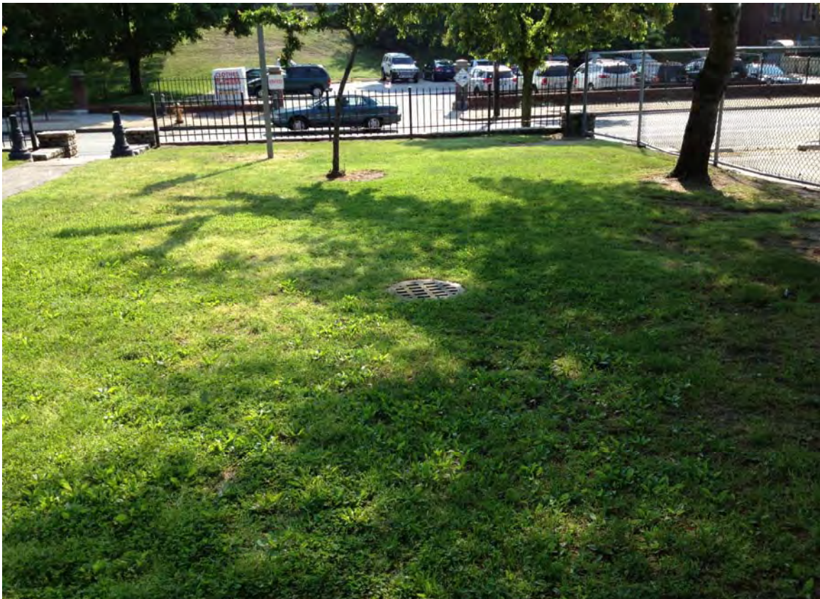
Catch basin at southeastern corner of property
