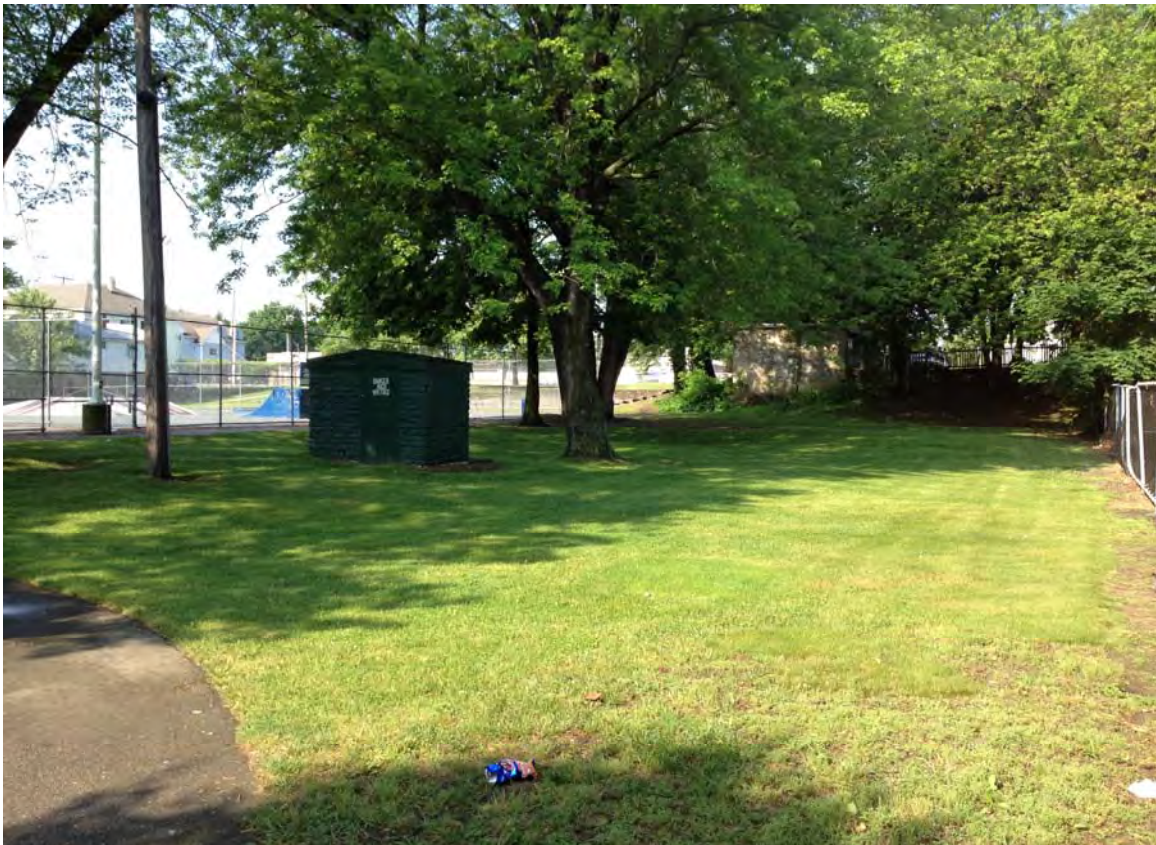
Utility pole and electrical building along northern edge of Site
