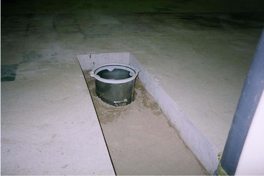
Extraction Well Vault Pre-pour
