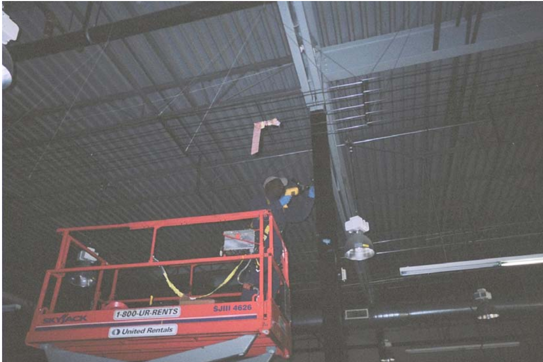
EW-7 Installation on Column
