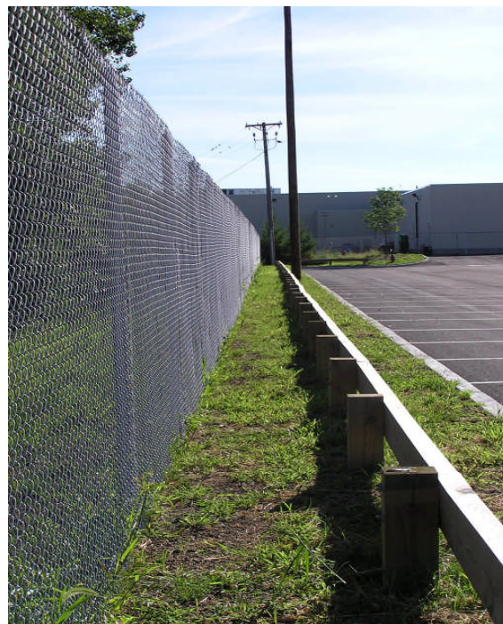
Photo 28: View of 8-ft. restrictive fencing installed on capped property parallel to the northern property line.
