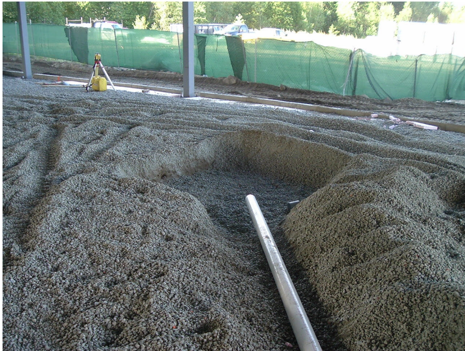
Photo 3: Typical suction pit progress photo illustrating early stage of construction.
