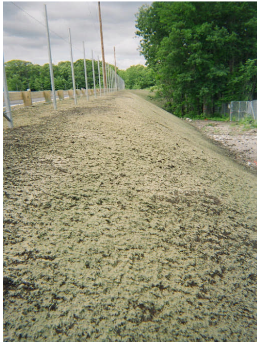
Photo 27: View of loamed and seeded cap along northern property line. Fence posts for restrictive fencing visible in upper left corner of the photo.
