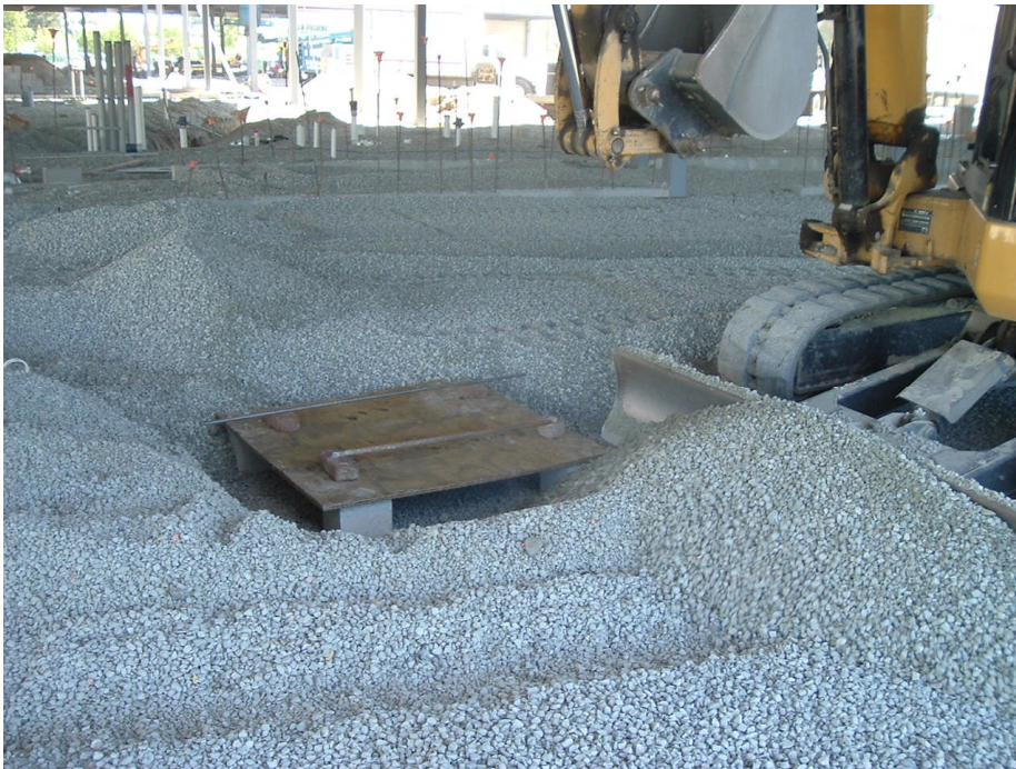
Photo 4: Typical suction pit progress photo illustrating middle stage of construction.
