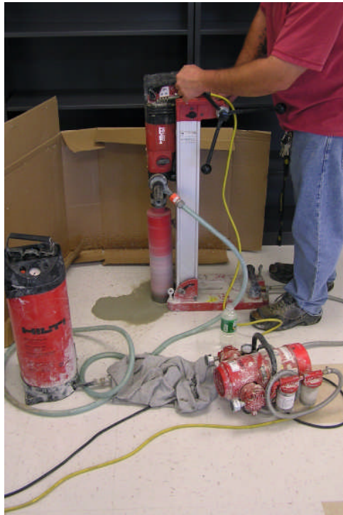
Photo 31: Progress photo of interior monitoring probe installation.
