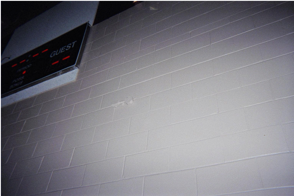
Photo 11: Typical view of interior sampling port located in gymnasium and cafeteria and connected to one of the continuous methane sensors.
