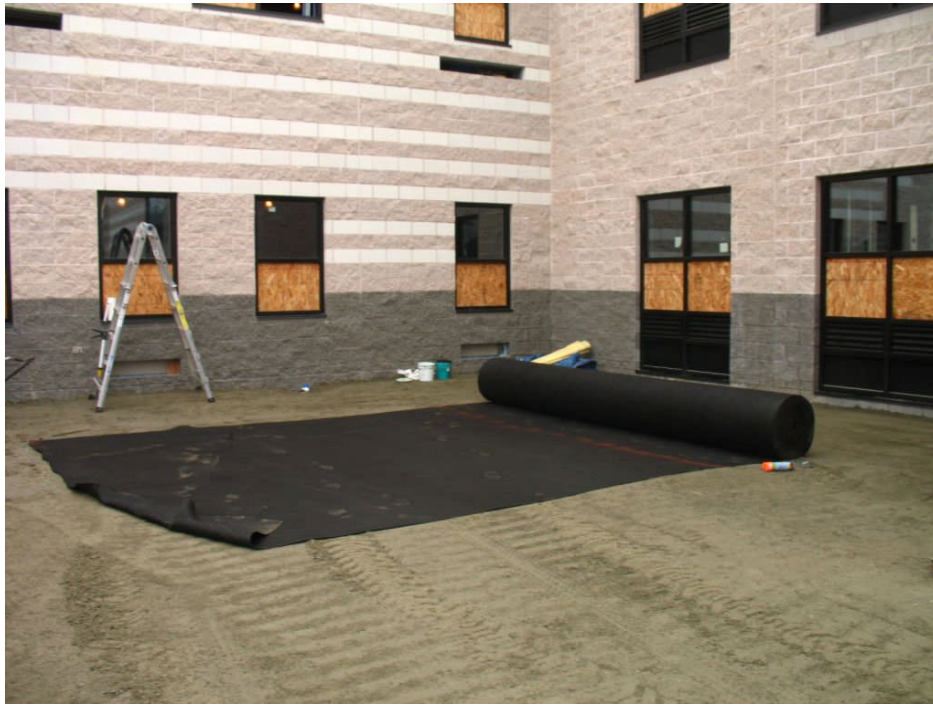
Photo 15: ProPex geotextile fabric being prepared for installation in future landscaped area.
