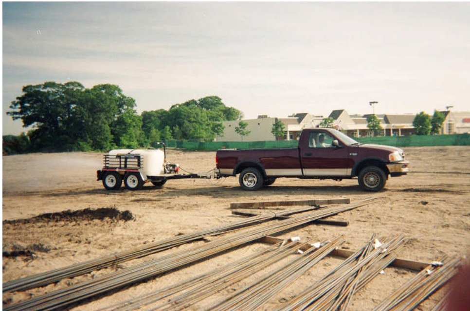
Photo 1: Water truck applying water for dust control at construction site.
