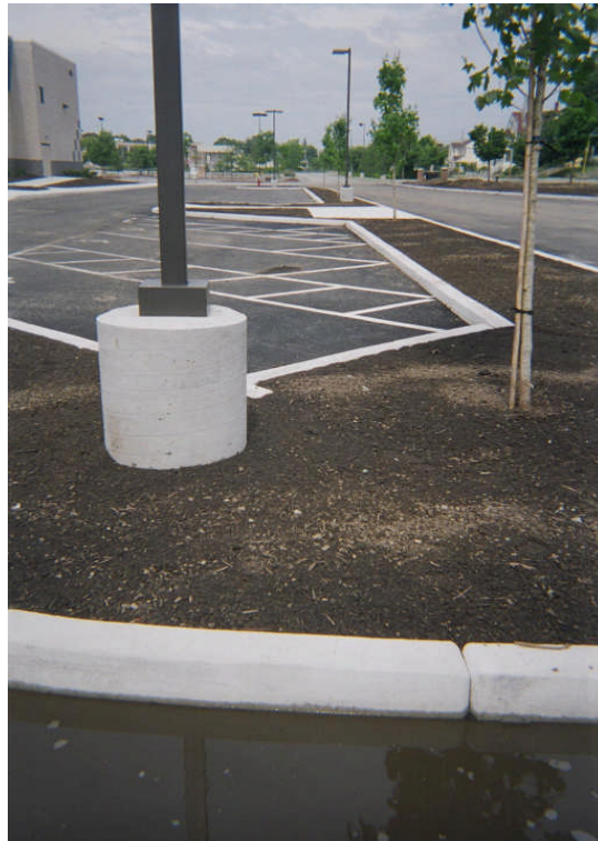
Photo 25: Cap completion photo illustrating loamed and landscaped parking island area and paved surfaces south of building.
