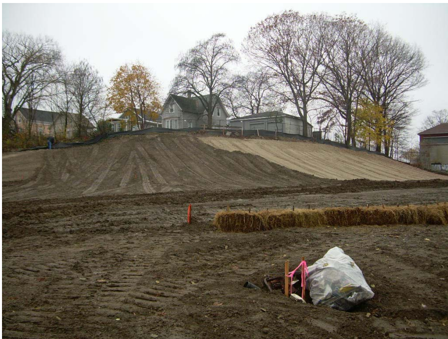
Photo 6: Continued installation of topsoil layer above sandy loam fill material.
