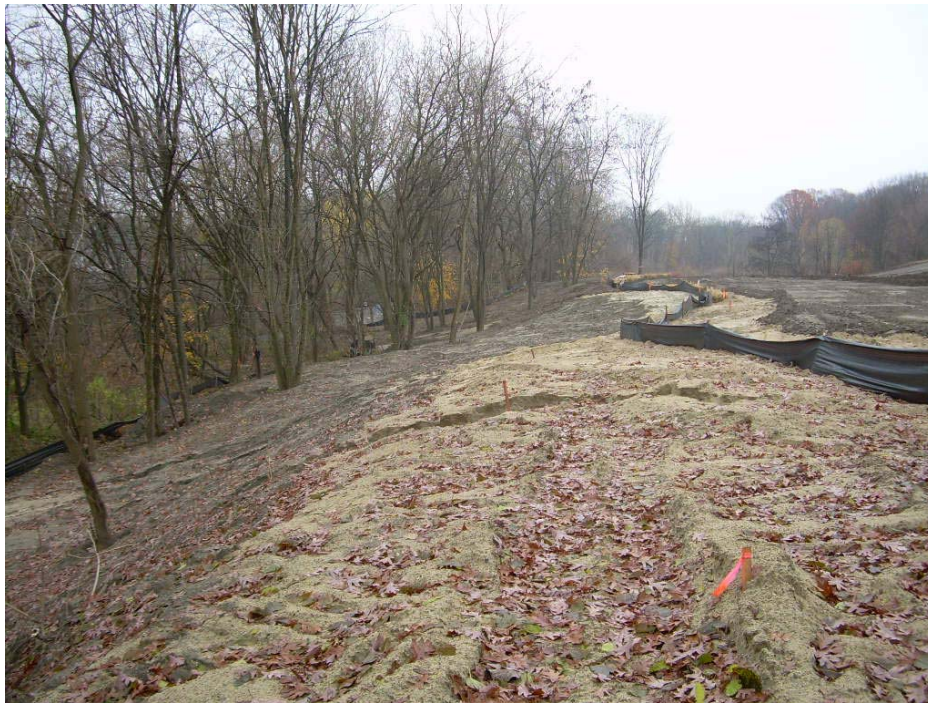
Photo 4: Transition zone between geotextile fabric and riparian restoration area.
