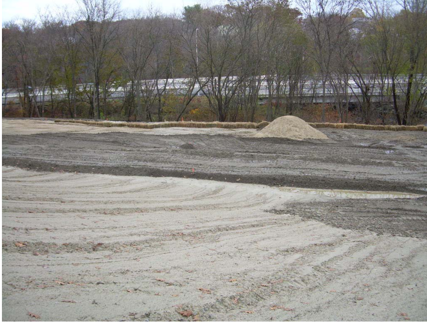
Photo 5: Installation of topsoil layer above sandy loam fill material.
