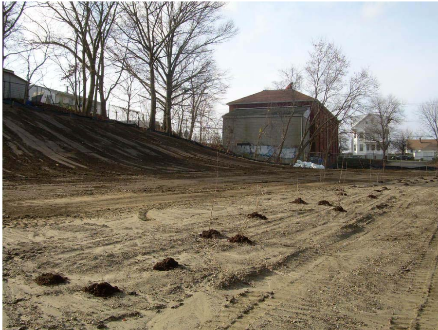
Photo 7: Installation of plantings along alignment of the future DOT bike path.
