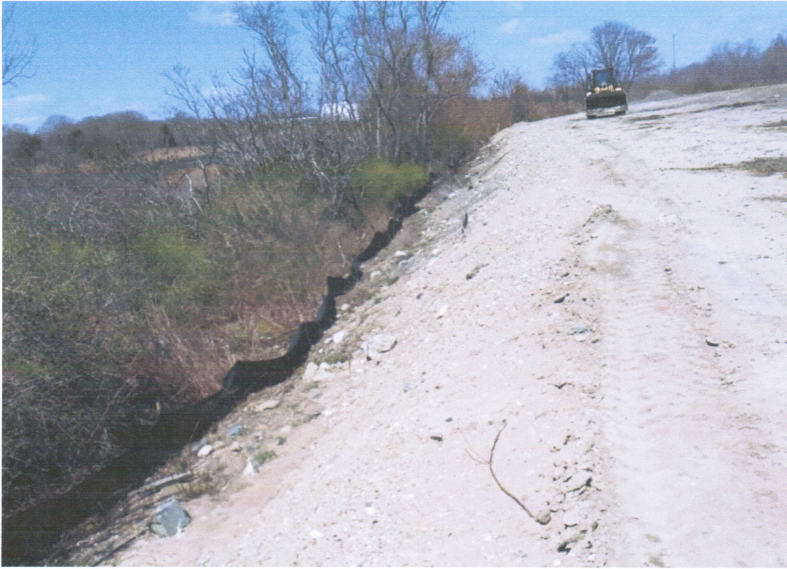
Photo 5 – Western Limit of Disturbance Looking North
