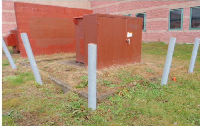
#3: Cavities around the electrical transformers behind the middle school.
