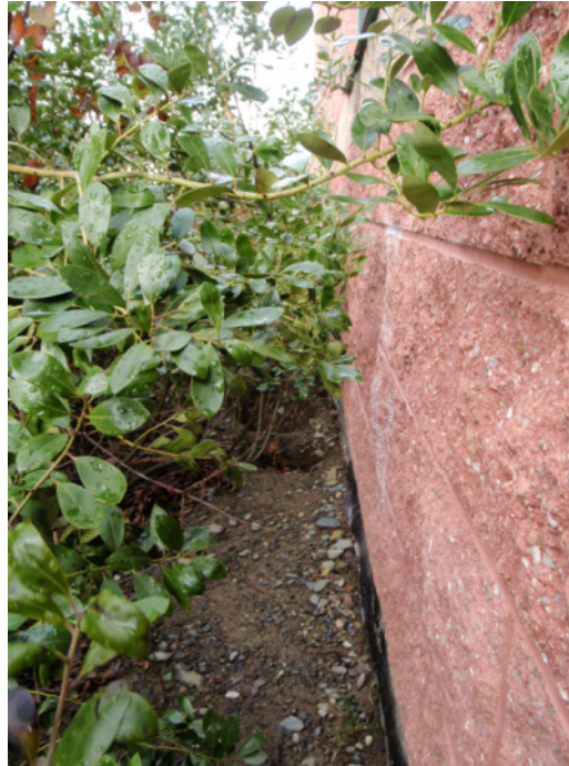
#1: Cavity behind a bush along the foundation in the courtyard area of the middle school.
