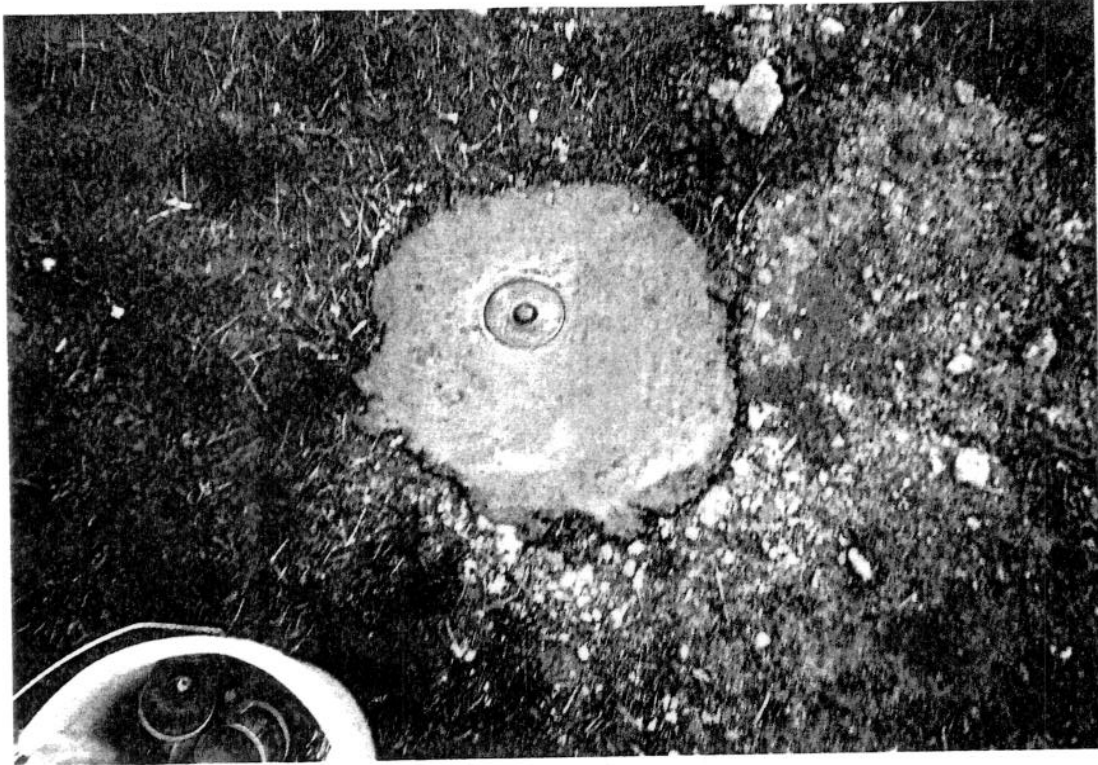
Monitoring Well WB-5 after repairs
