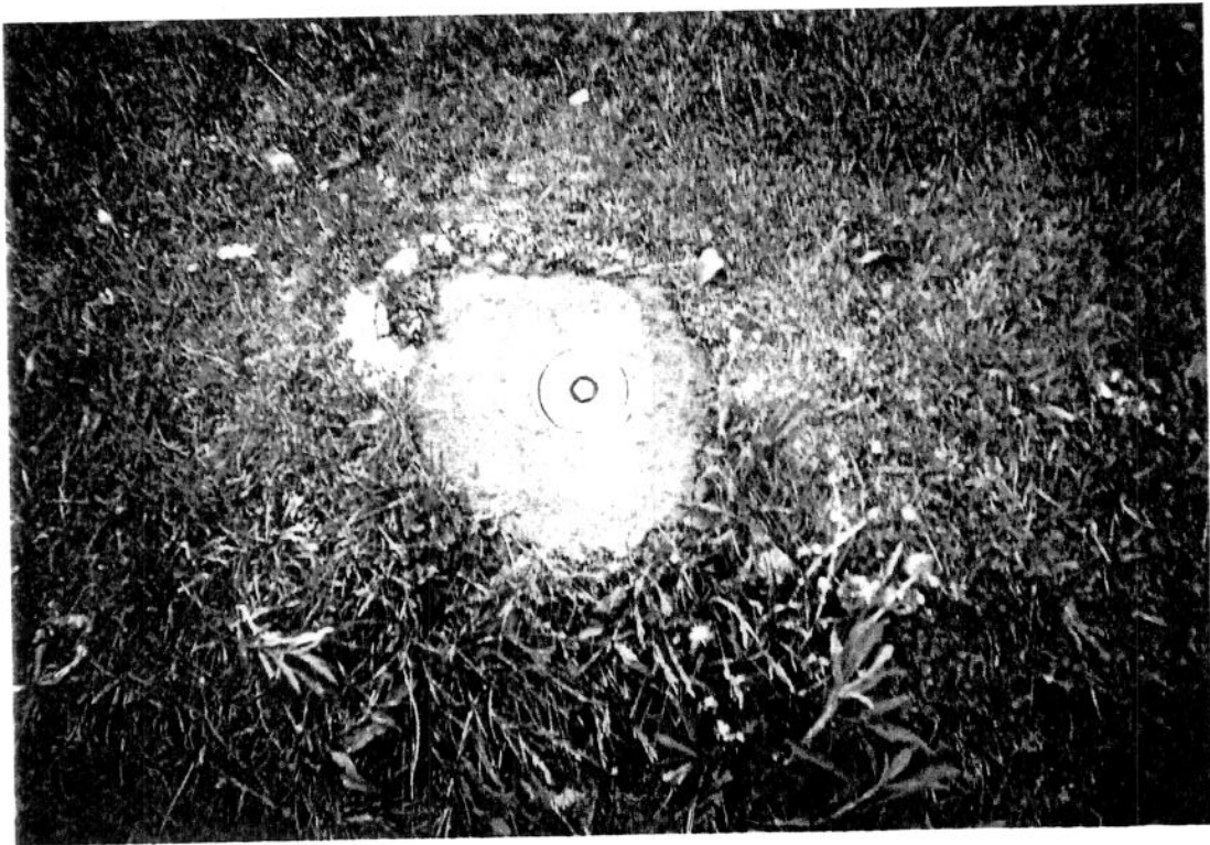
Monitoring Well WB-13 after repairs
