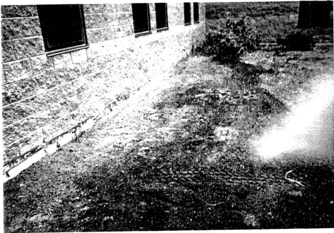
Photograph 12. South wall of middle school courtyard
