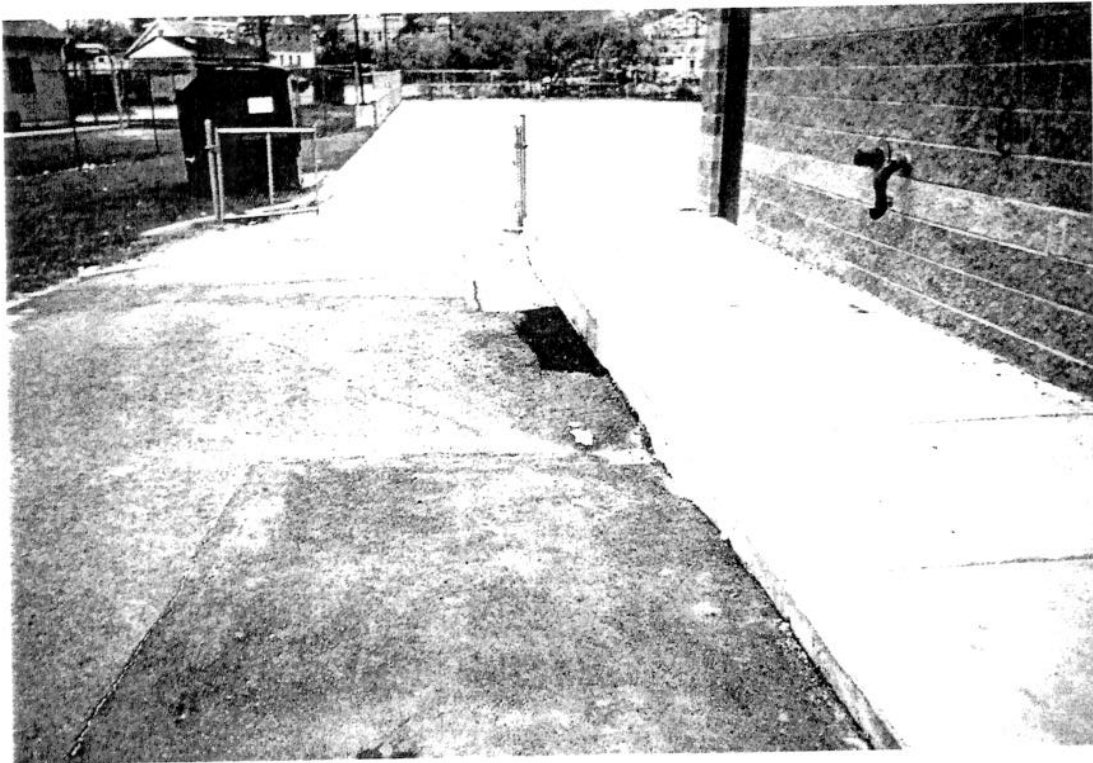
Photograph 6. Northwest wall of middle school gym
