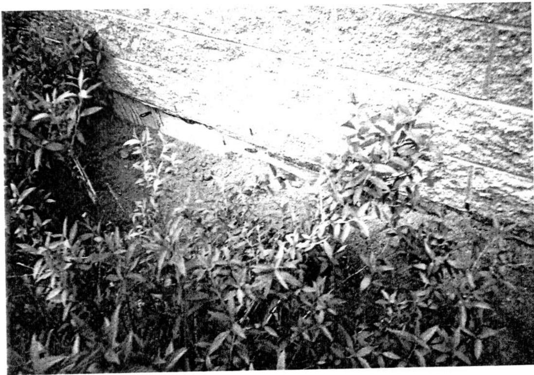
Photograph 8. Eastern wall of middle school courtyard
