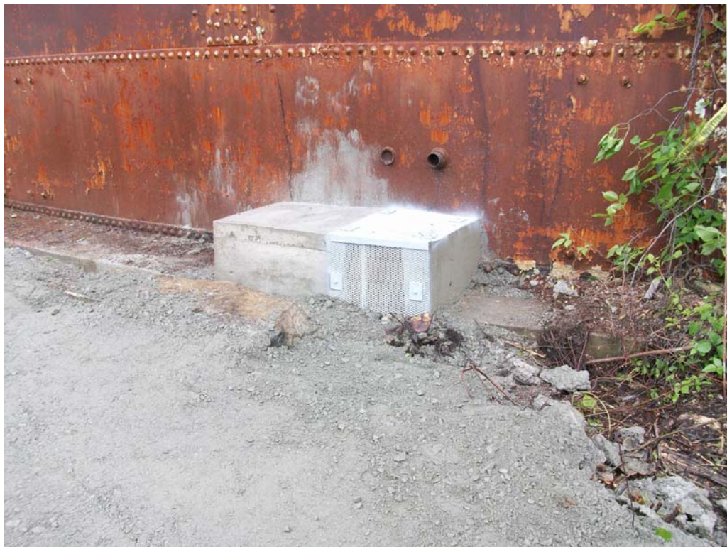
Photo 2: Pipe Stub Encased in Concrete and Steel Grate Valve Protection
