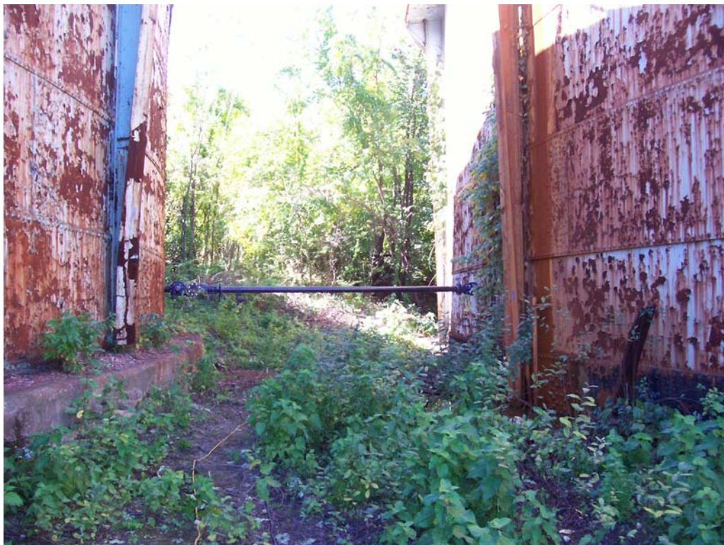
Photo 4: Gas Holder Connection Line Installed in October 2009
