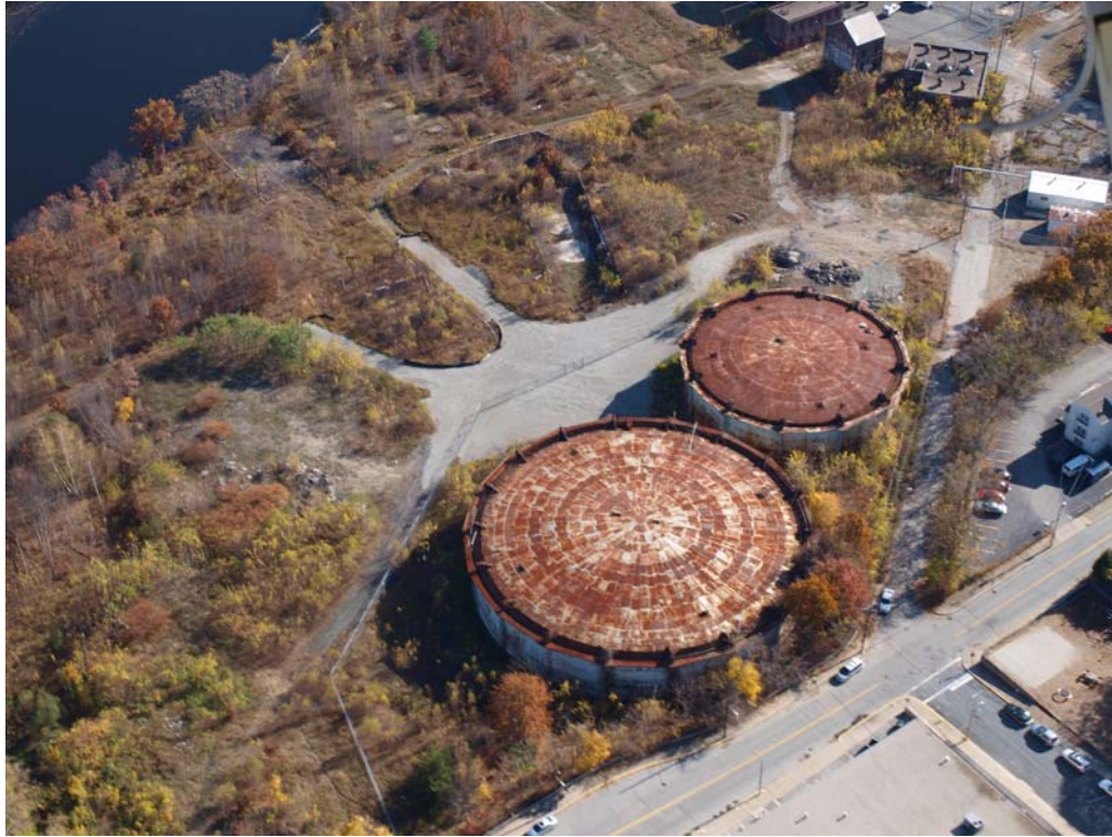
Photo 3: Gas Holders and Restored Area
