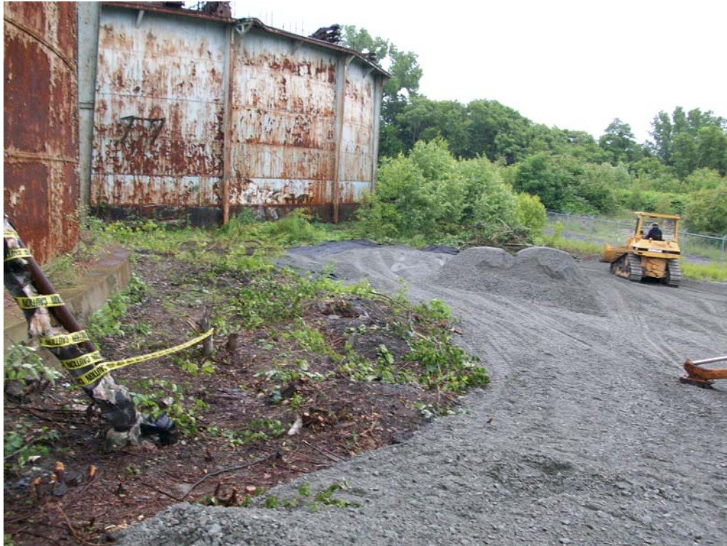
Photo 1: DGCS and Filter Fabric Installation
