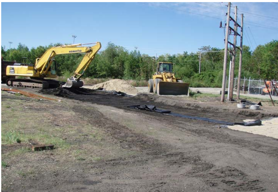
Photo No. 10 - T-Ford excavating roadway/parking areas in May 2010.
