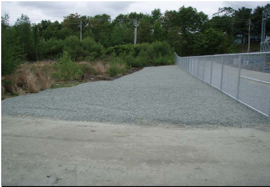
Photo No. 17 - Finished extended low lying area cap.
