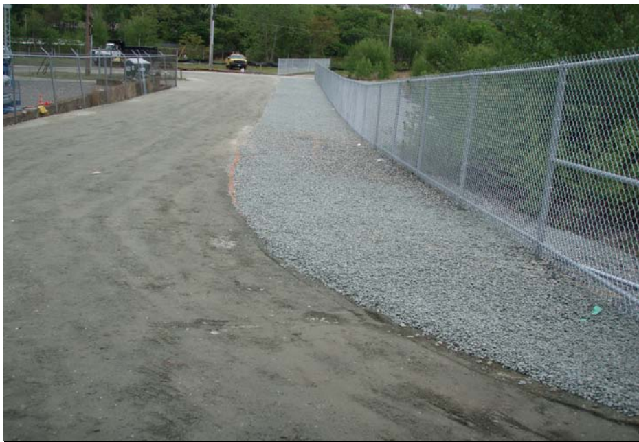
Photo No. 14 - Finished roadway and low lying area cap with fence.
