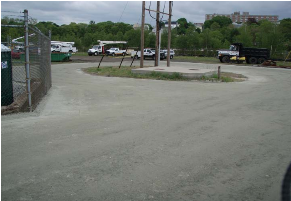
Photo No. 15 - Finished roadway and parking area cap.
