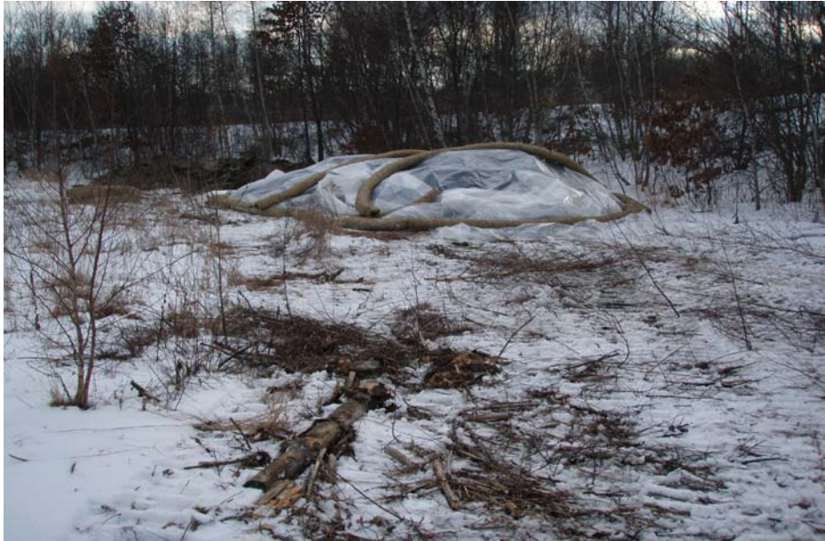
Photo No. 7 - Segregated stockpile of blue-stained material located in soil relocation area (January 2010). Material placed on and covered with polyethylene sheeting.
