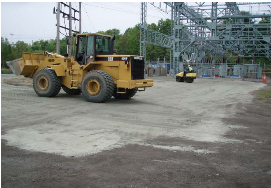
Photo No. 12 - T-Ford grading and compacting roadway (May 2010).
