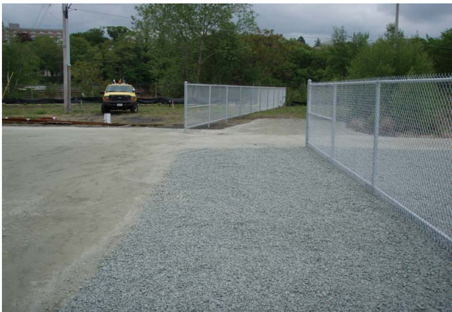
Photo No. 16 - Finished roadway and low lying area cap and fence.
