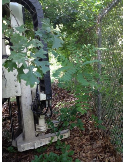
Photo 2 – Geoprobe Rig During Installation
