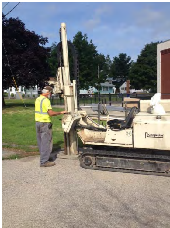
Photograph No. 31 Installation of SVP-11S with the geoprobe direct push rig.
