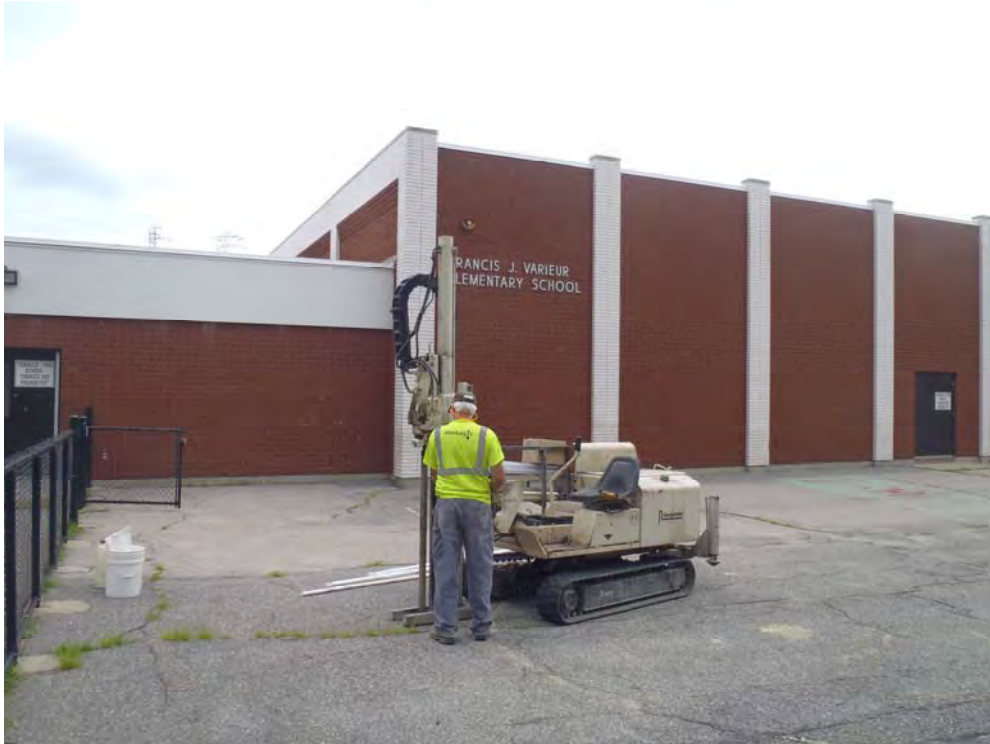
Photograph No. 30 Installation of SVP-13S with a geoprobe direct push rig.
