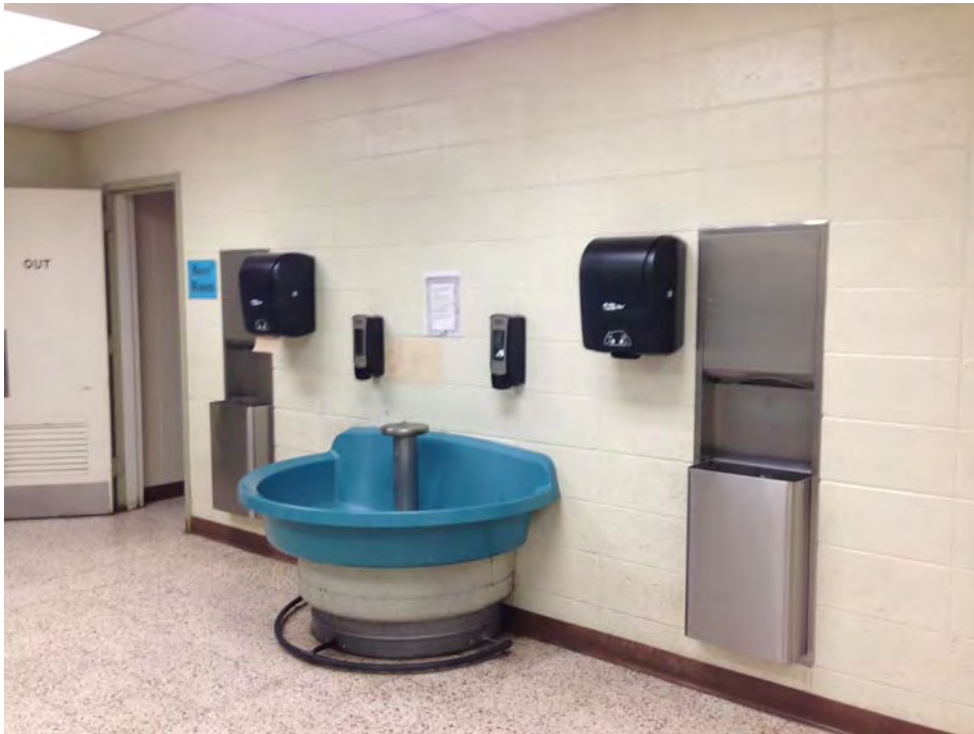
Photograph No. 9 Sink outside of the gymnasium/cafeteria.
