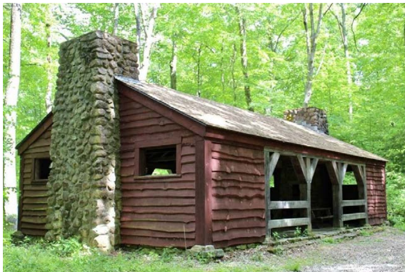
Picnic shelter constructed by DFE and the Appalachian Mountain Club at the backpack campsite. Photo credit: Megan Ruggieri
