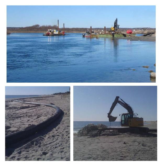
A hydraulic cutter head suction dredge working at the Ninigret Pond sedimentation basin in Charlestown, RI (top center), and pipe laid along the beach used to pump sediment (bottom left) from the dredge vessel for disposal on Charlestown Town Beach (bottom right). (Pictures taken by Eric Schneider, DFW)
