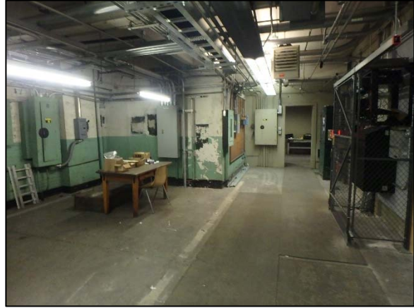
Photo 10 Overview of the northern portion of the main switchboard room located on the second floor on September 9, 2018, as viewed from the southeast.
