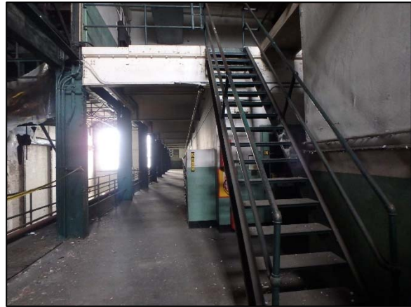
Photo 12 Overview of the mezzanine located on the fourth floor on September 9, 2018, as viewed from the north.
