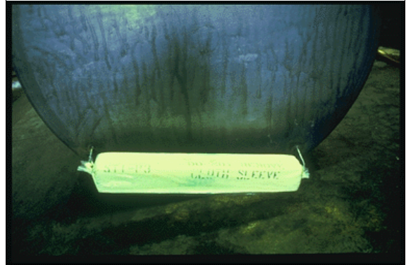
Sample Galvanic (or sacrificial) anode
