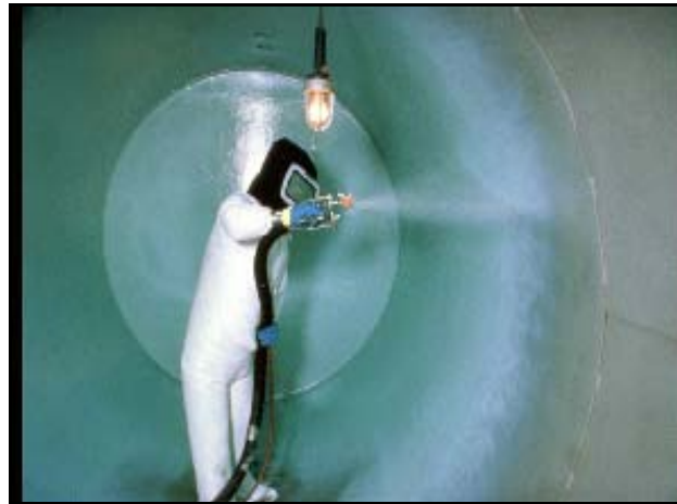
Sample of a Tank being Interior Lined
