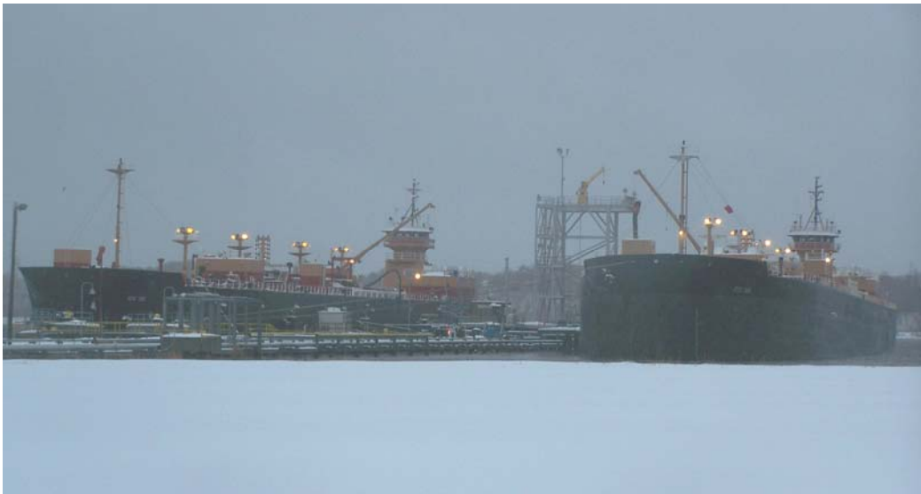
Figure 13. Reconstructed dock returned to service; simultaneously accepting deliveries from a barge and a coastal tanker.
