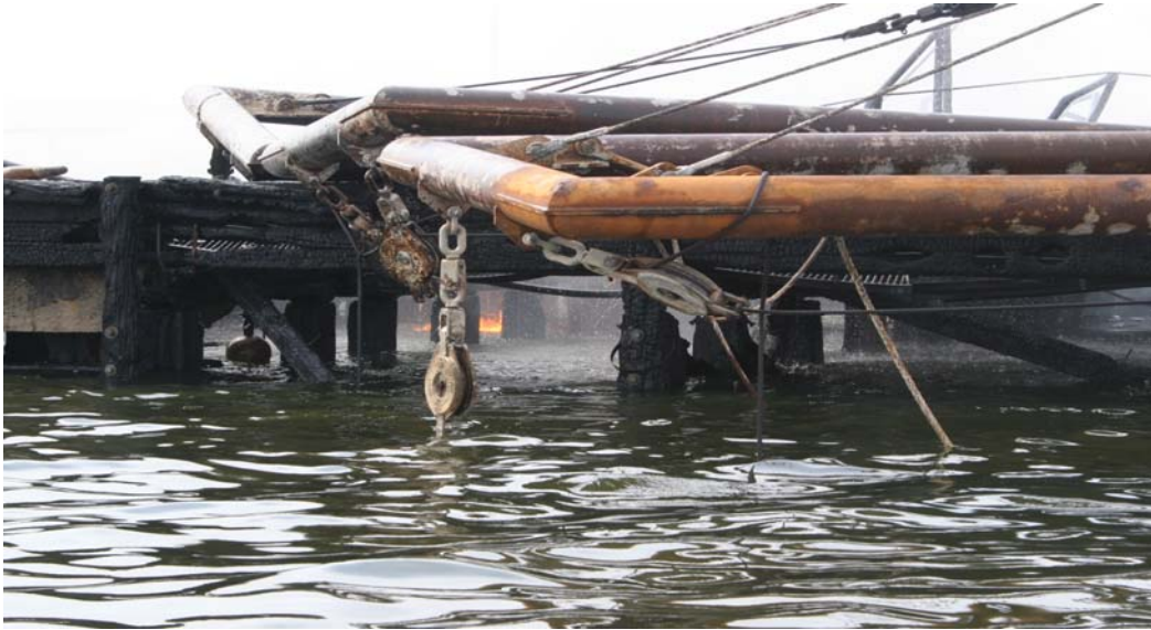
Figure 11. Collapsed transfer gantry; fires from burning piers and ruptured product lines.
