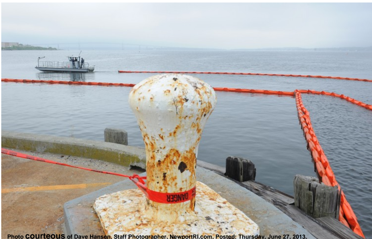
Figure 5. Naval Station Newport Port Operations personnel place a second boom around the west end of Pier 1 during a mock oil spill emergency response drill on Thursday.
