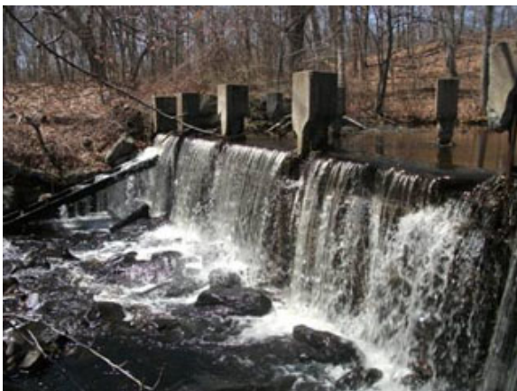
Shady Lea dam removal in North Kingstown
