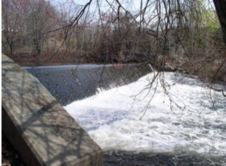
Manton Pond Dam fishway construction in Johnston
