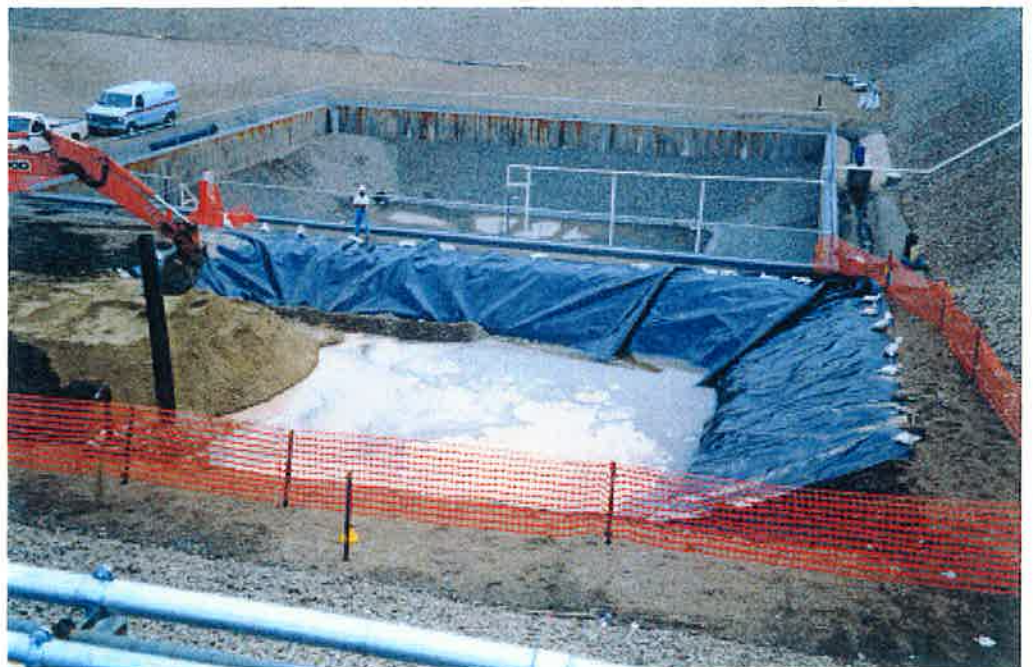
Backfill operations in SALNG Area within the dike.
