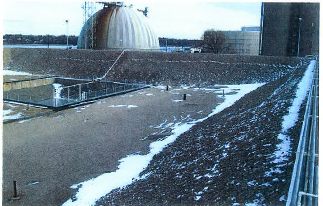
View of recent conditions of SALNG within the containment dike.
