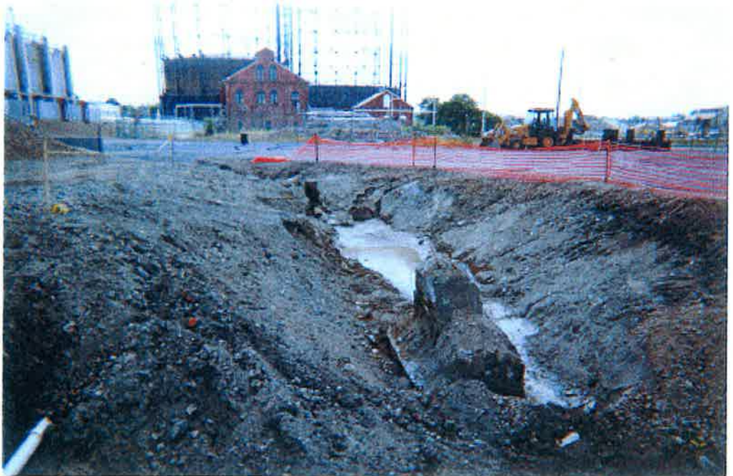
View of pipe trench excavation looking westerly.
