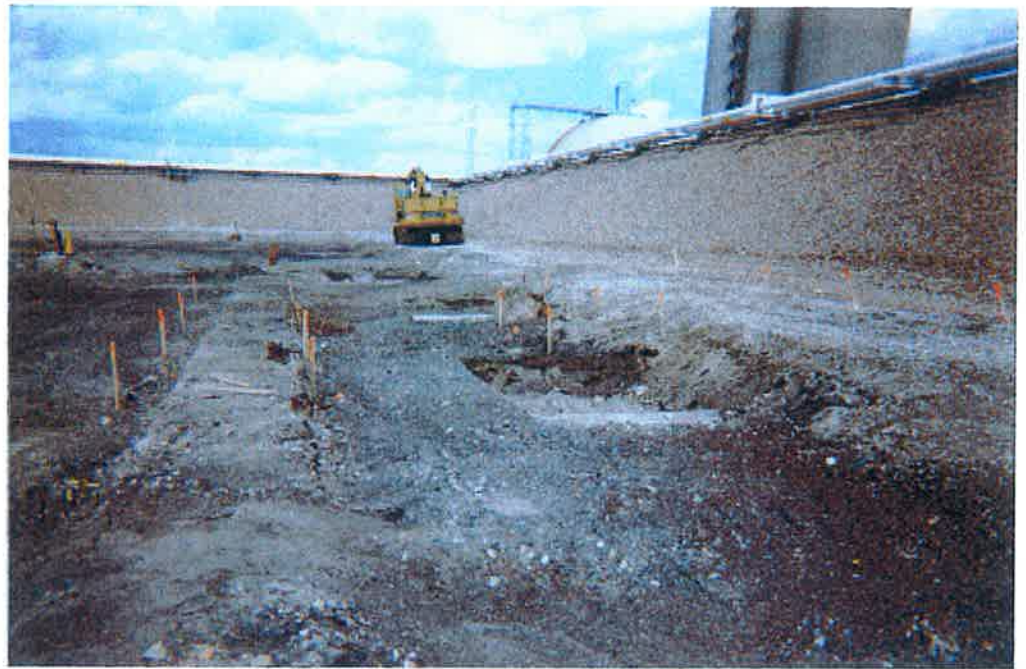
View of southeast corner of SALNG excavation.
