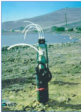
Landfill site over fractured granite, monitored with five Waterloo Systems. Each System comprised of dedicated Double Valve Pumps and Pressure Transducers in 4-6 intervals to depths of 275 feet (84m). The Multi-Purge Manifold allowed the monitoring of 21 zones to be completed in less than 2 days.
