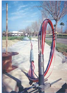
Contaminant investigation at a U.S. Air Force Base. Waterloo Systems installed to 700 ft. in overburden using screened and cased wells. Up to 6 zones per hole with dedicated pumps and transducers.
