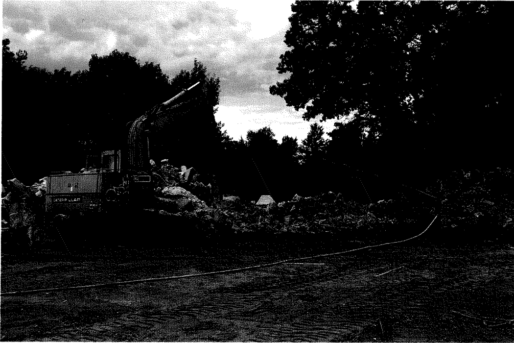
PHOTO 1 – Water being applied to concrete crushing prep, for dust control
