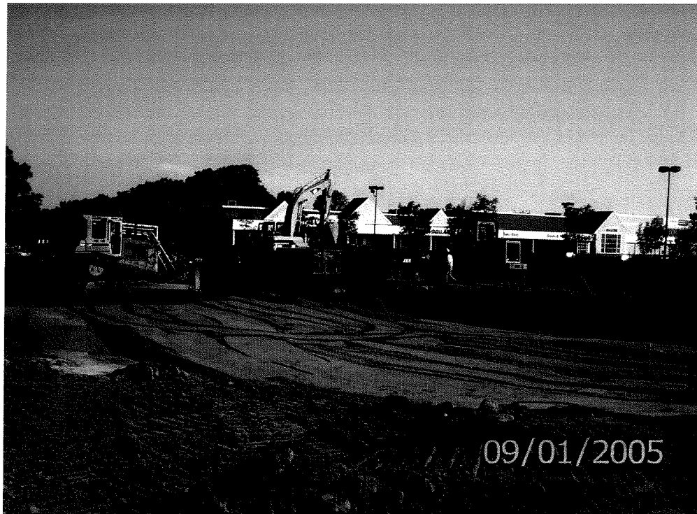
PHOTO 6 – General photo of bulldozer working material into excavation
