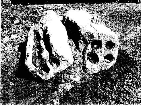
13. Transite pipes encased in concrete.
