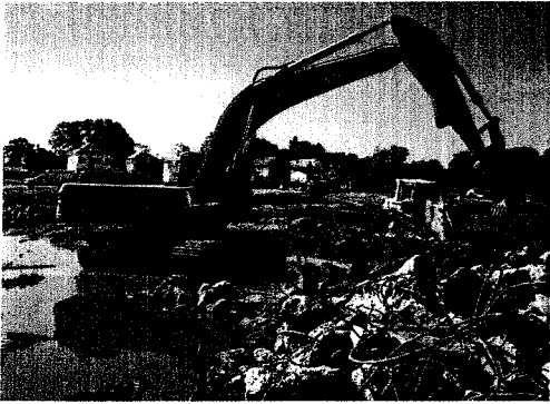
15. Separating foundation from re-bar.
