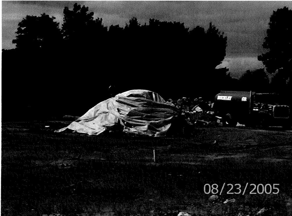
PHOTO 5 – 6 Mil poly to cover stockpile created from excavation
