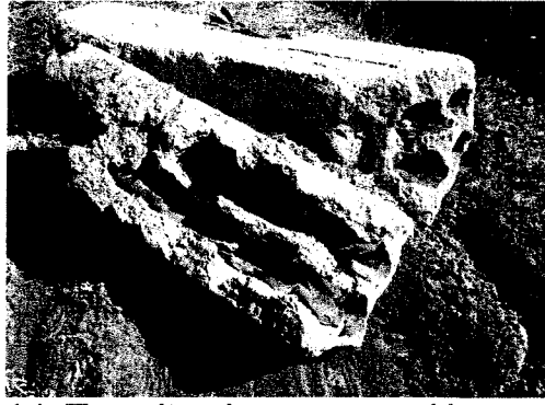
14. Transite pipes encased in concrete.
