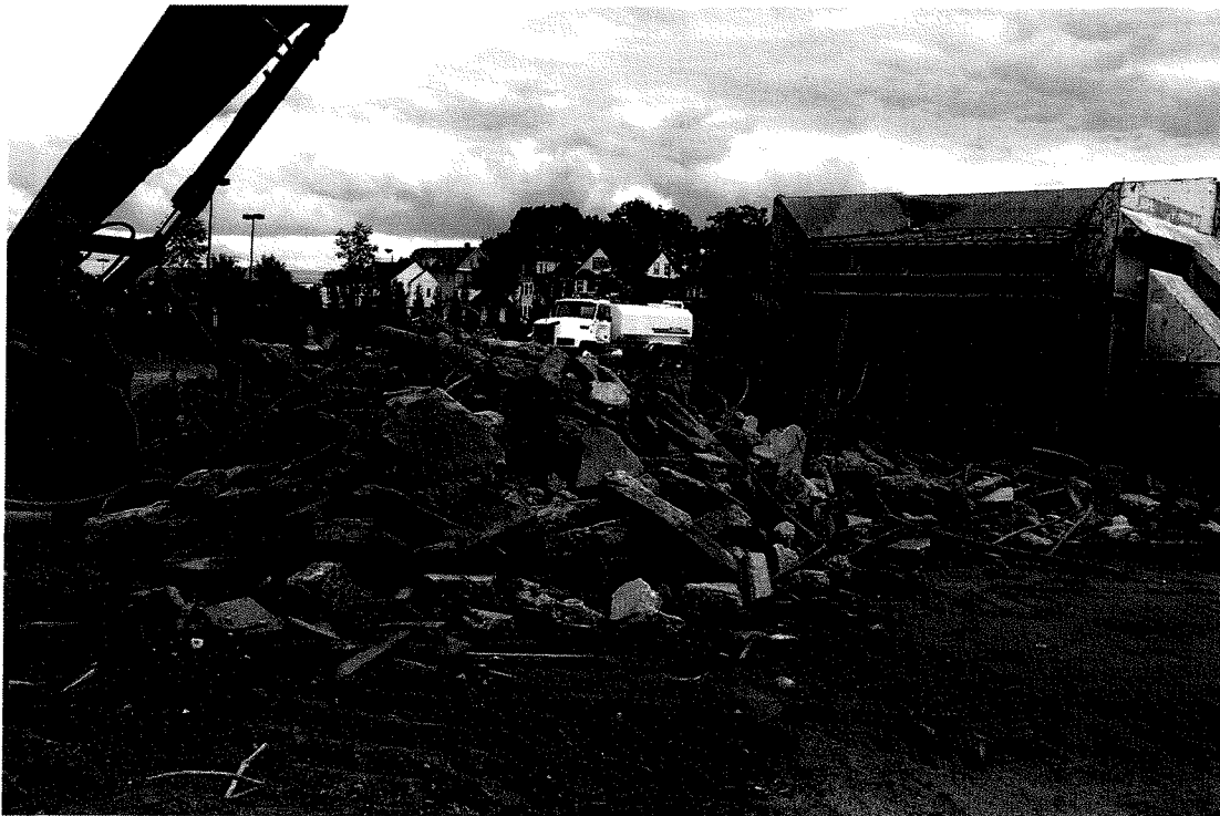
PHOTO 4 – General photo of concrete, wood and metal debris screened out of existing material
