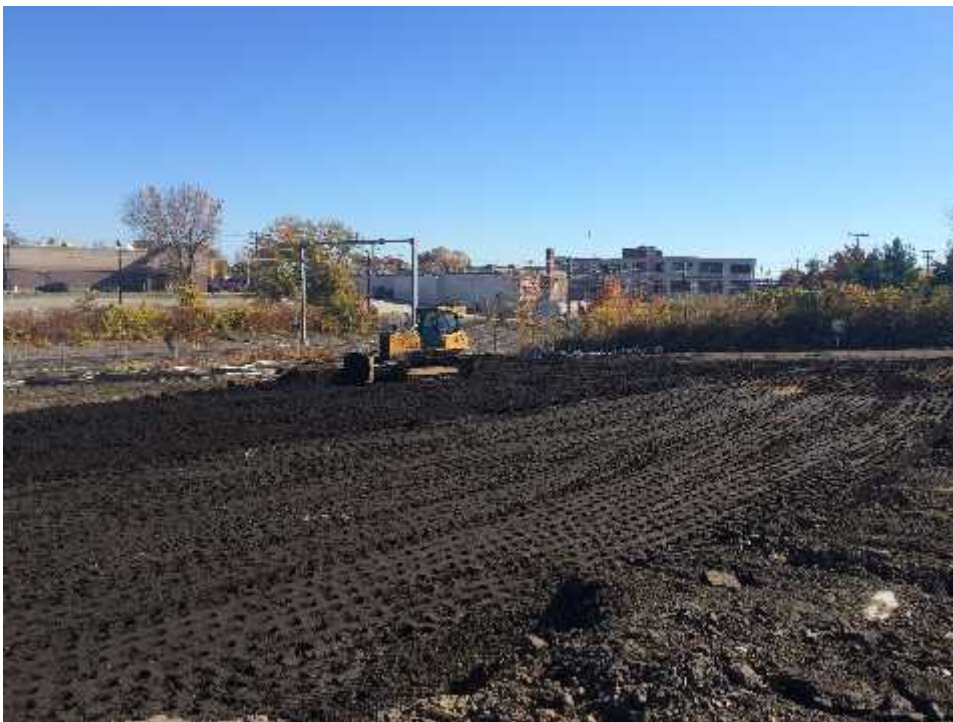
Photo 30 Capping of Inner Cove sediments in Carriage House Area
