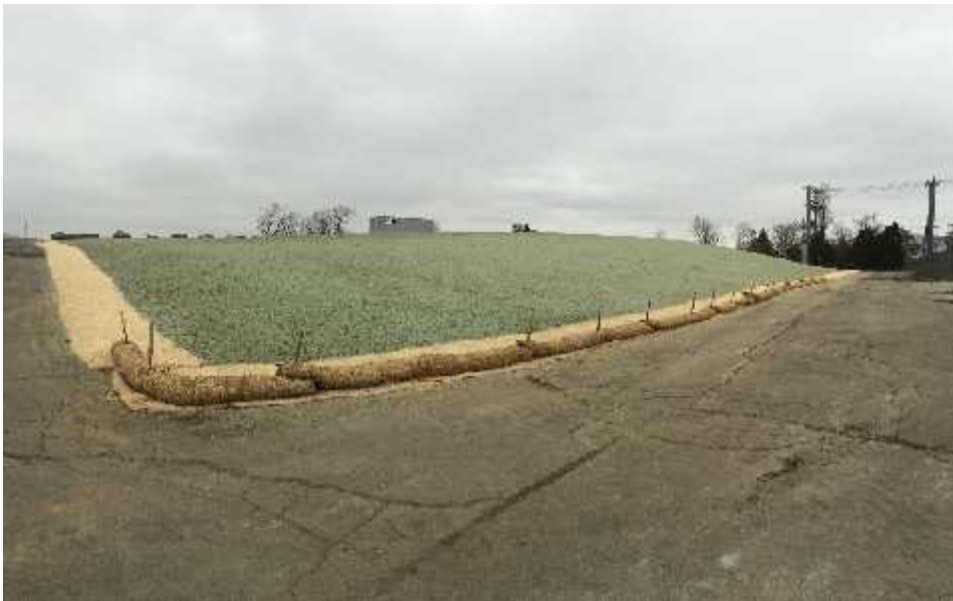
Photo 34 Phase III, sediment area, final grades with hydroseed
