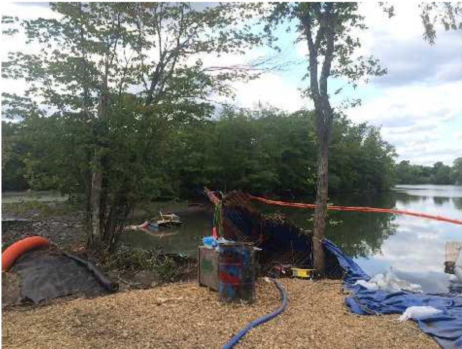
Photo 6 Inner Cove initial dewatering
