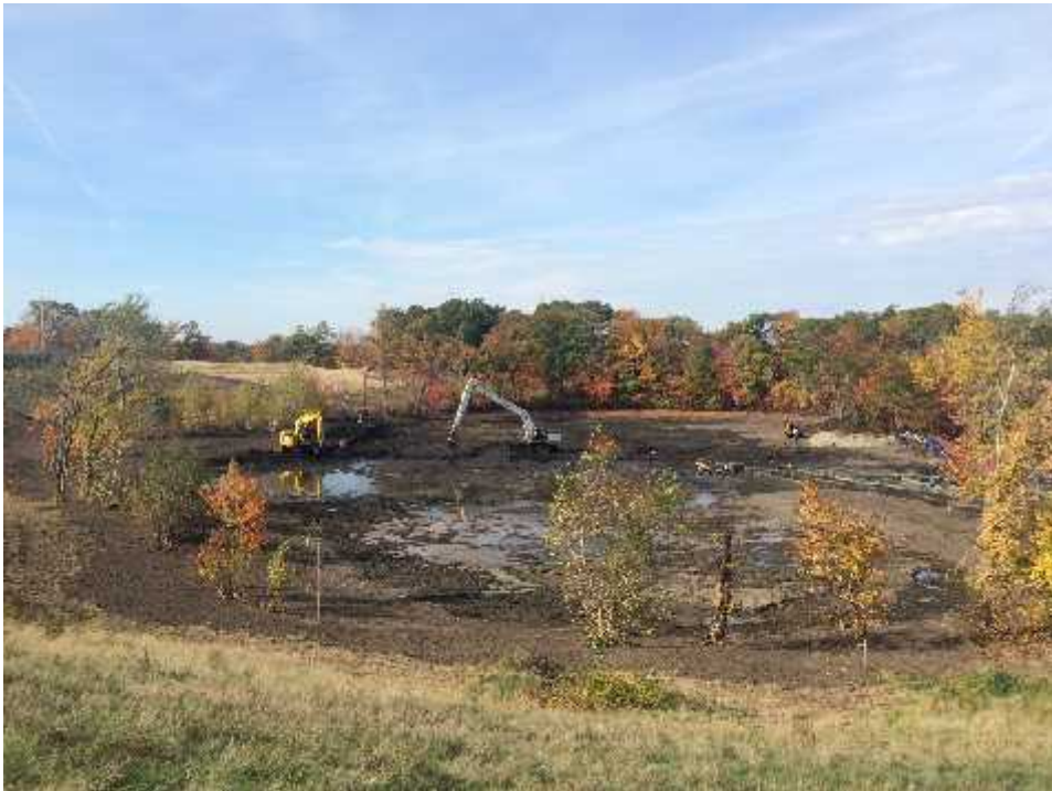
Photo 16 Inner Cove cap installation
