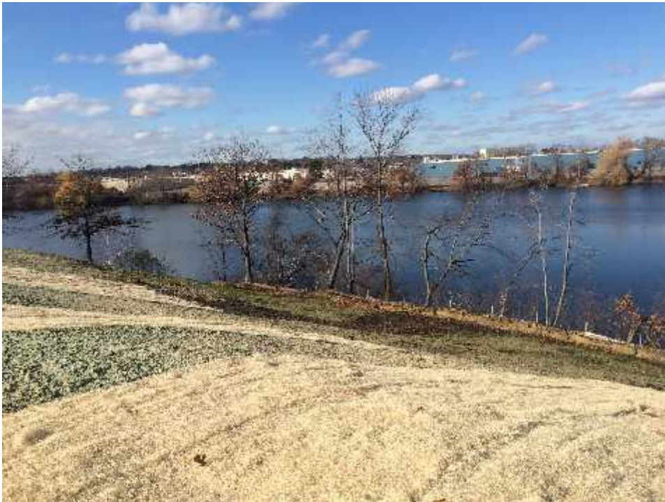
Photo 32 Completed Phase III with hydroseed and erosion control matting
