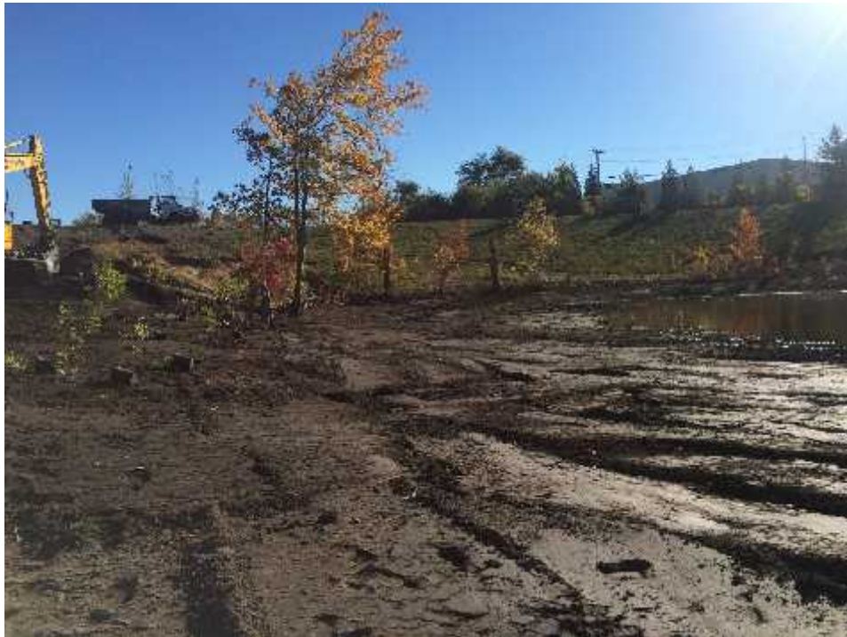
Photo 18 Inner Cove cap and wetland restoration
