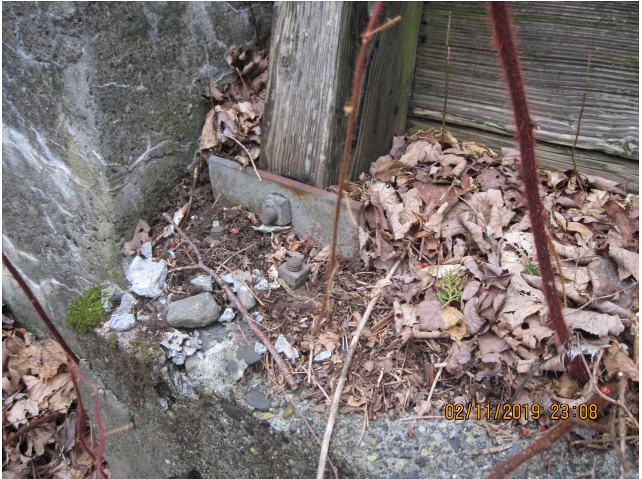
Photo #4: Typical Wall Anchorage to Foundation
