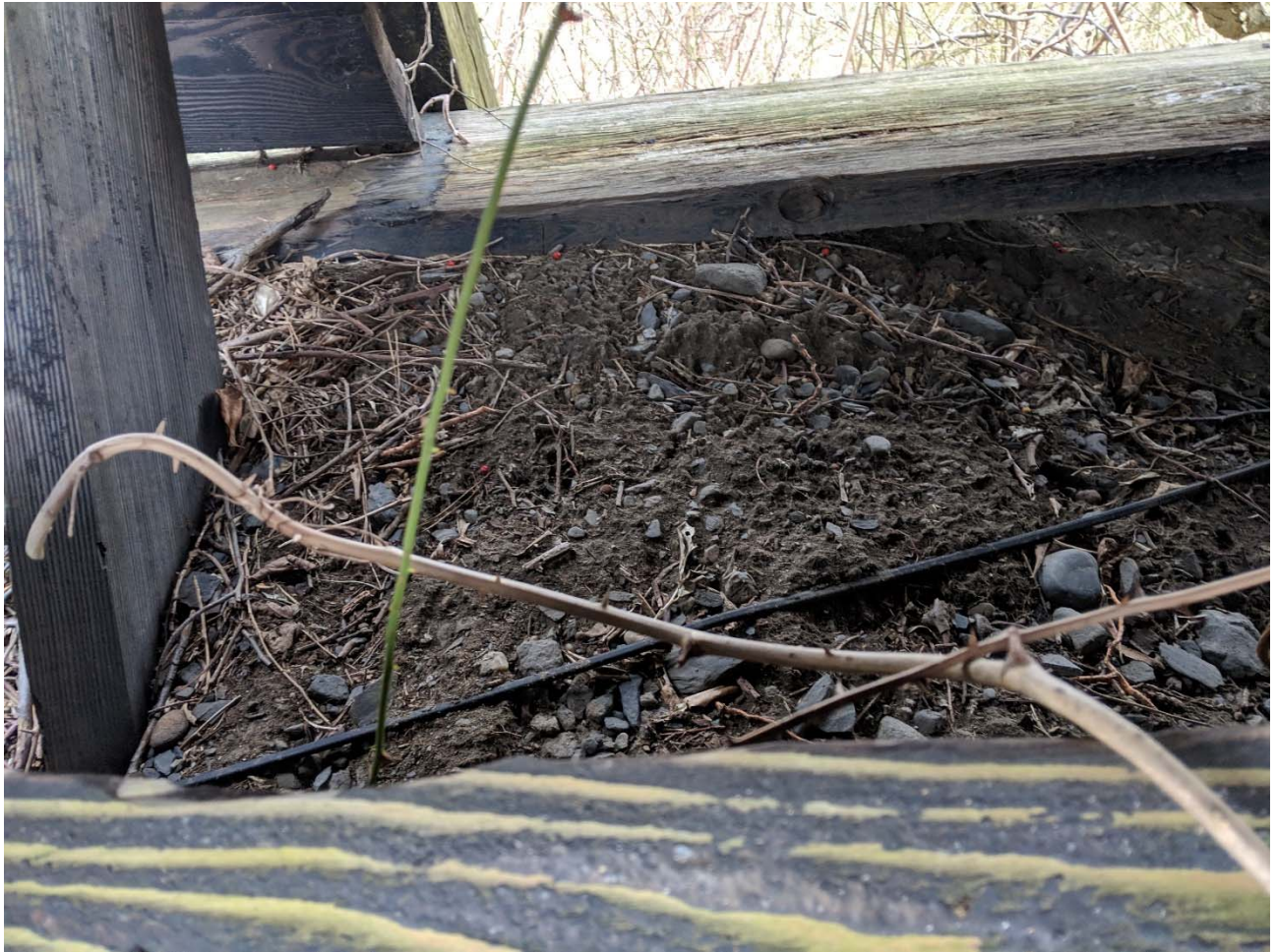
Photo #3: View of Earthen Fill Within Wall
