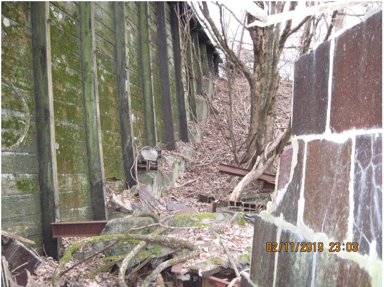
Photo #1: View of West side of Wall
