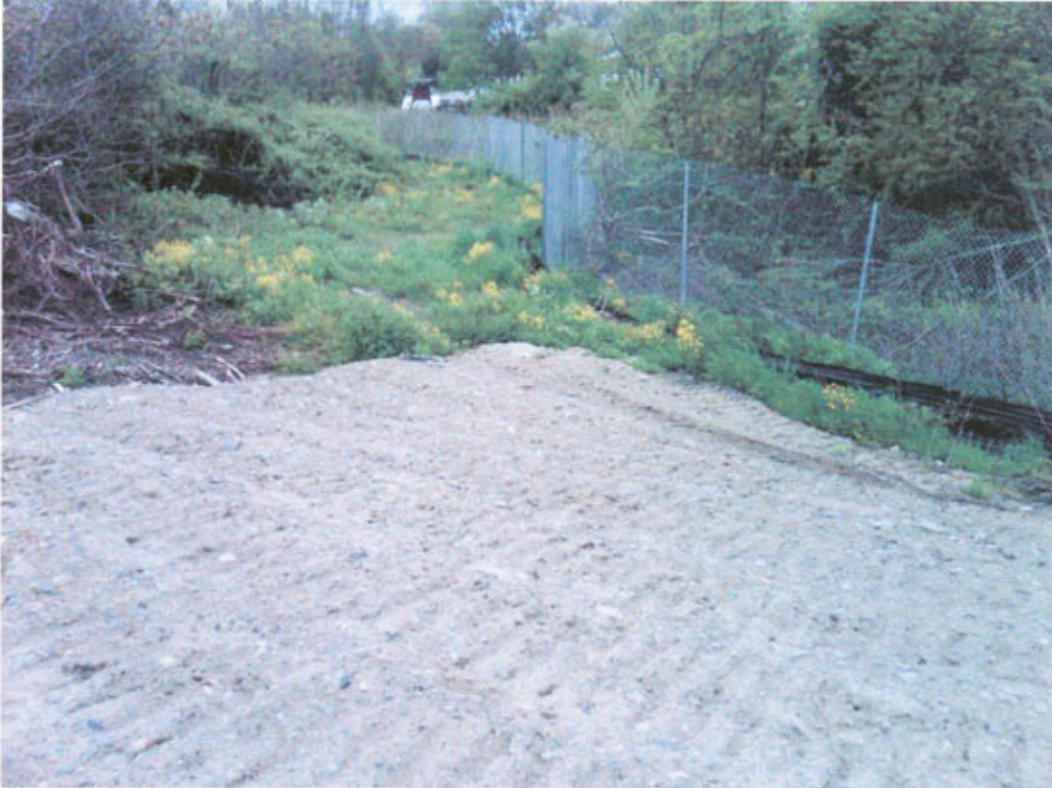
Photo 2 – Erosion Control and Fencing along Northern Property Line
