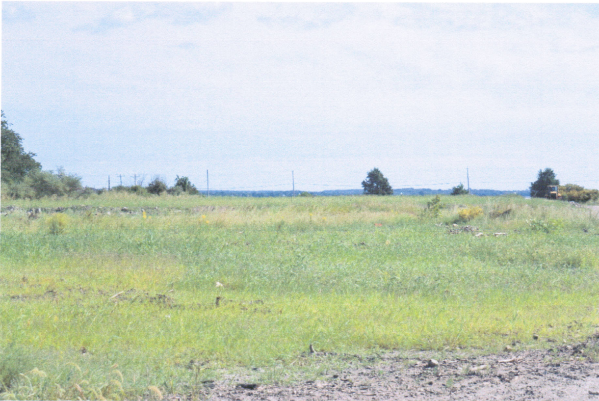
Photo 2 – Central Portion of Landfill Looking South
