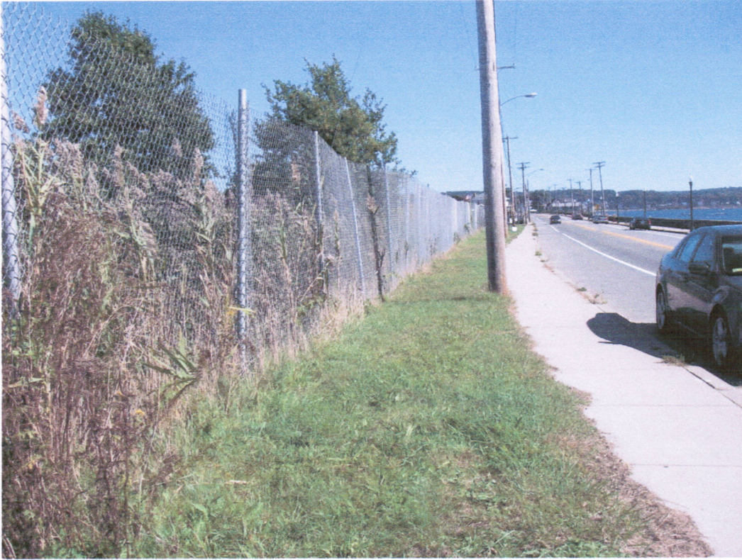
Photo 1 – Along the Southern (Park Avenue) Limit of Disturbance
