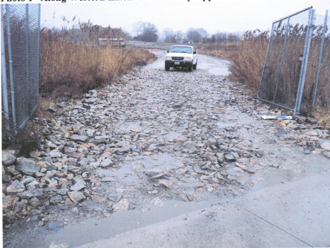
Photo 2 – At Park Avenue Gate
