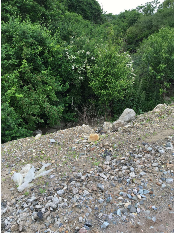
Photo 3 : Erosion on the western slope
