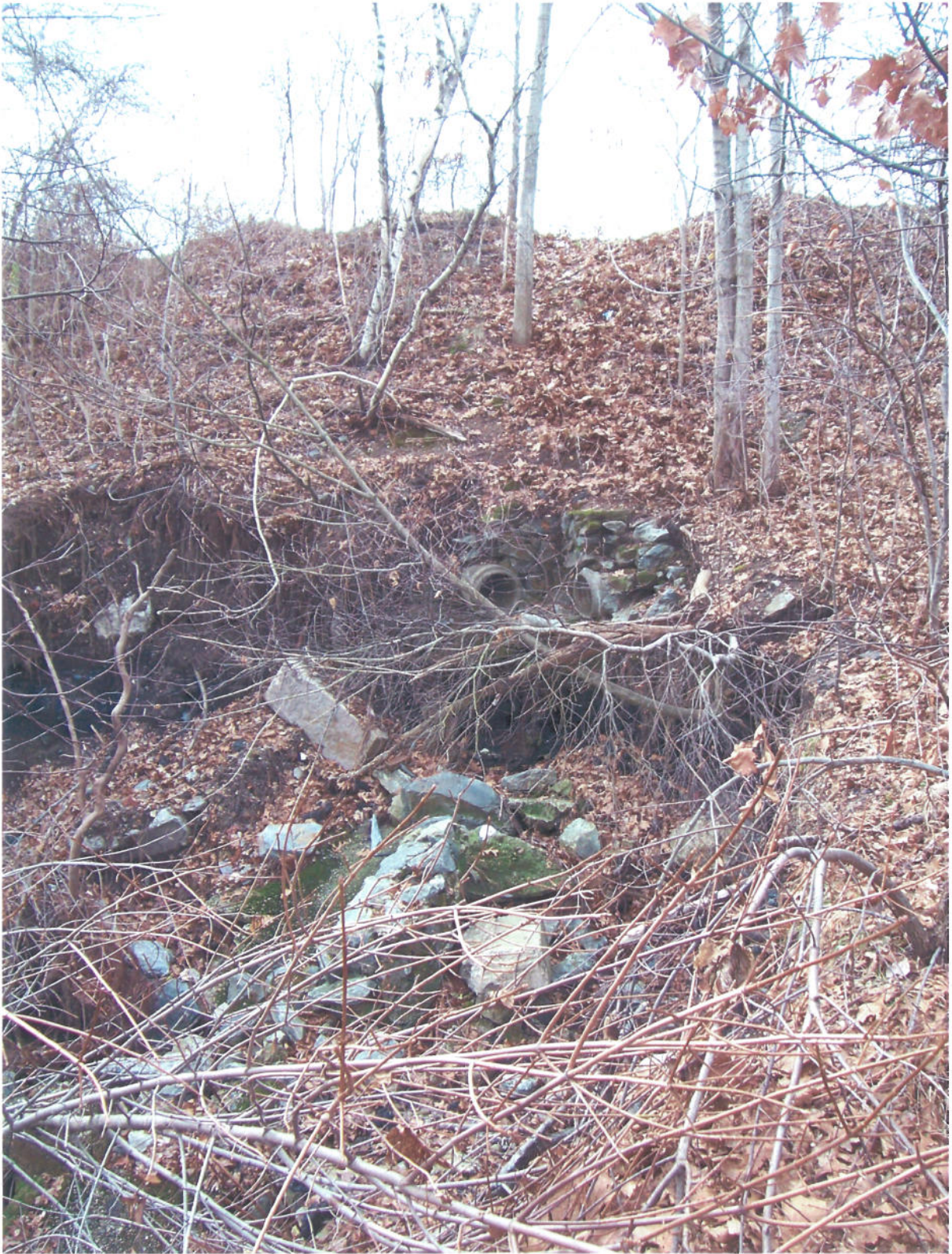
Photo 1 View of South Washout Area. Two drain lines visible in distance.
