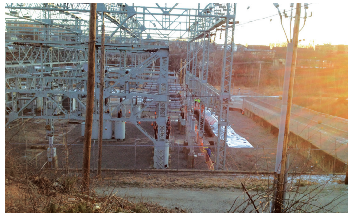
The majority of excavation associated with upgrading the existing Tidewater electrical substation is complete.
