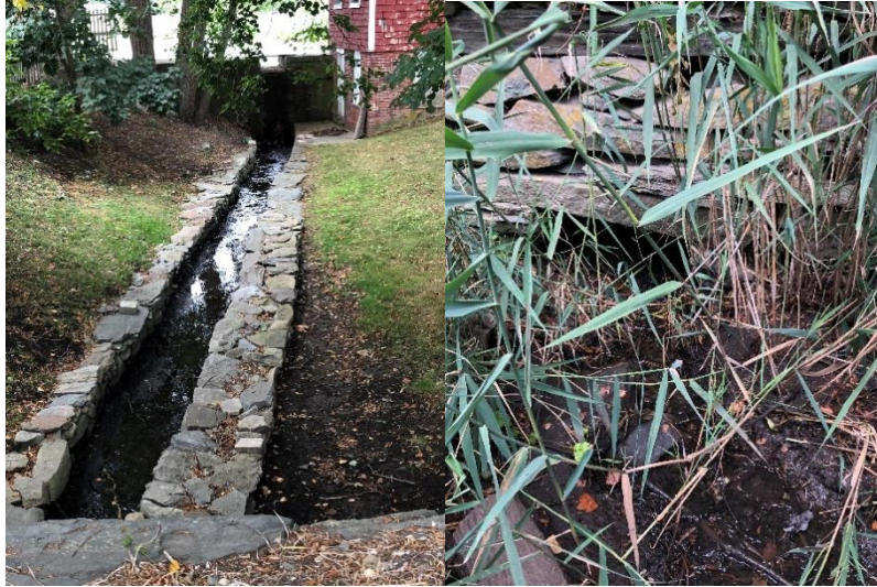
Figure 5: Source 2020-5-007 a small stream exiting a grazing pasture that is bound by a concrete trench (left) and exits to the growing area through a retaining wall (right).
