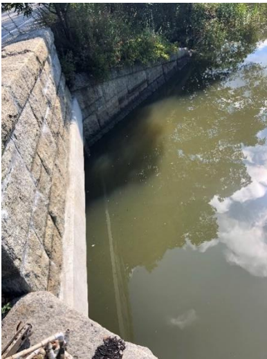
Figure 4: source 2020-5-001 flow over dammed reservoir at Kickemuit Reservoir.
