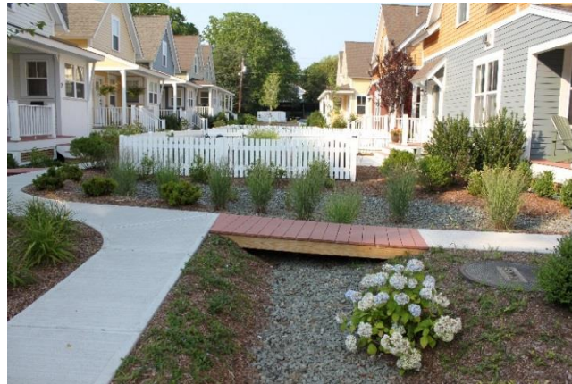
Cottages on Greene - bioretention, bioswales, and permeable pavement in compact cottage development in East Greenwich.
