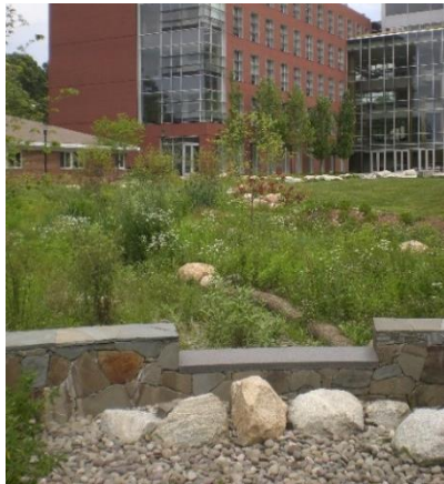
Large bioretention area on the University of Rhode Island Kingston campus to offset impervious surface created by the Center for Biotechnology and Life Sciences building.
