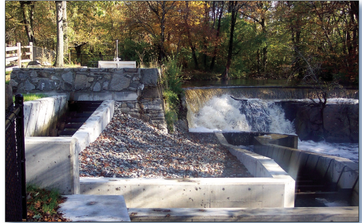
Figure 3. A fish ladder, completed in 2012, bypasses Hunt's Mill Dam on the Ten Mile River.
