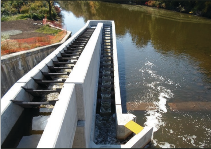
Figure 2. A fish ladder was installed to bypass the Turner Reservoir Dam in 2012.
