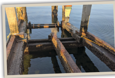
Rotted framing timber removal.
