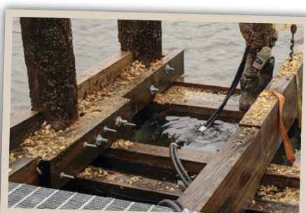
New timber and grating installation
