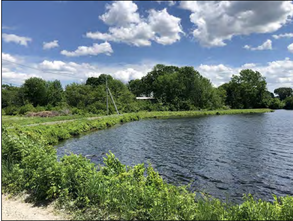
Photo No. 47: Pine Ledge Road to West Greenville Road Dam – Upstream side of the embankment from pine ledge road looking right.
