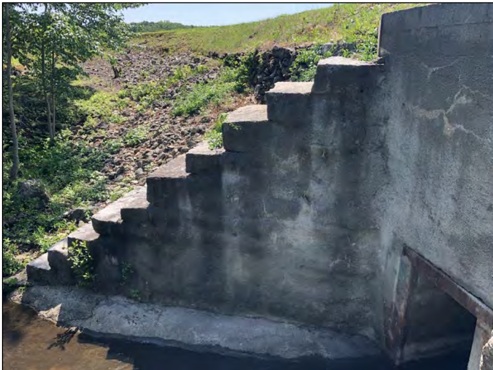
Photo No. 20: Main Dam - The outlet right downstream channel wall.
