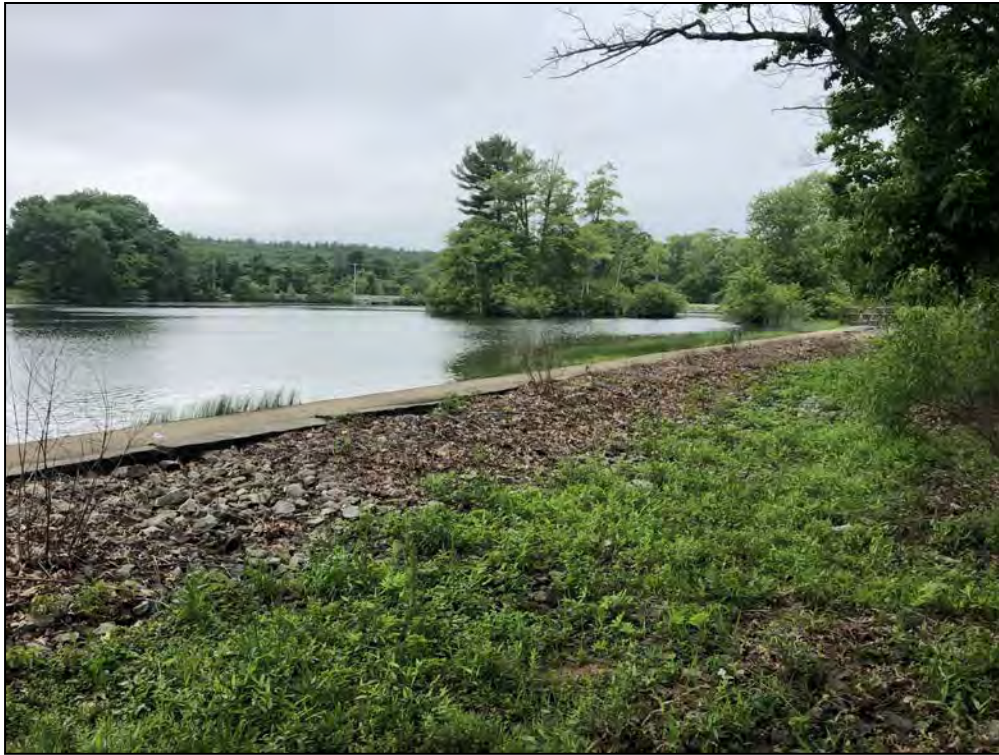
Photo No. 67 Spillway Section – Discharge area of the spillway.
