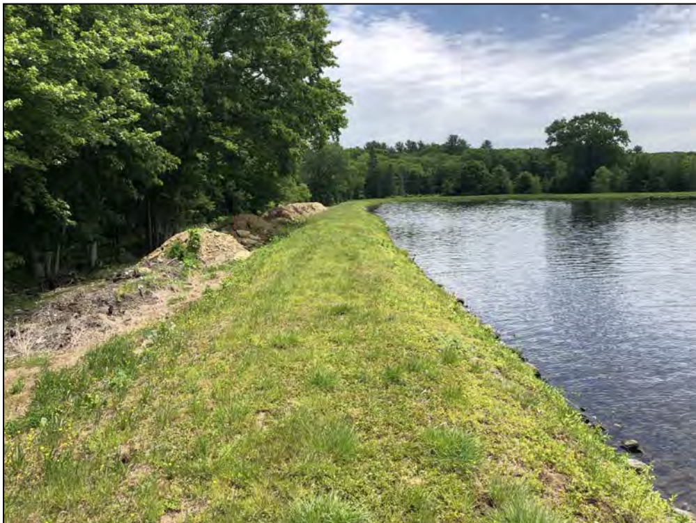
Photo No. 28: Bookers Dam - Crest from near STA 12+00 looking right.
