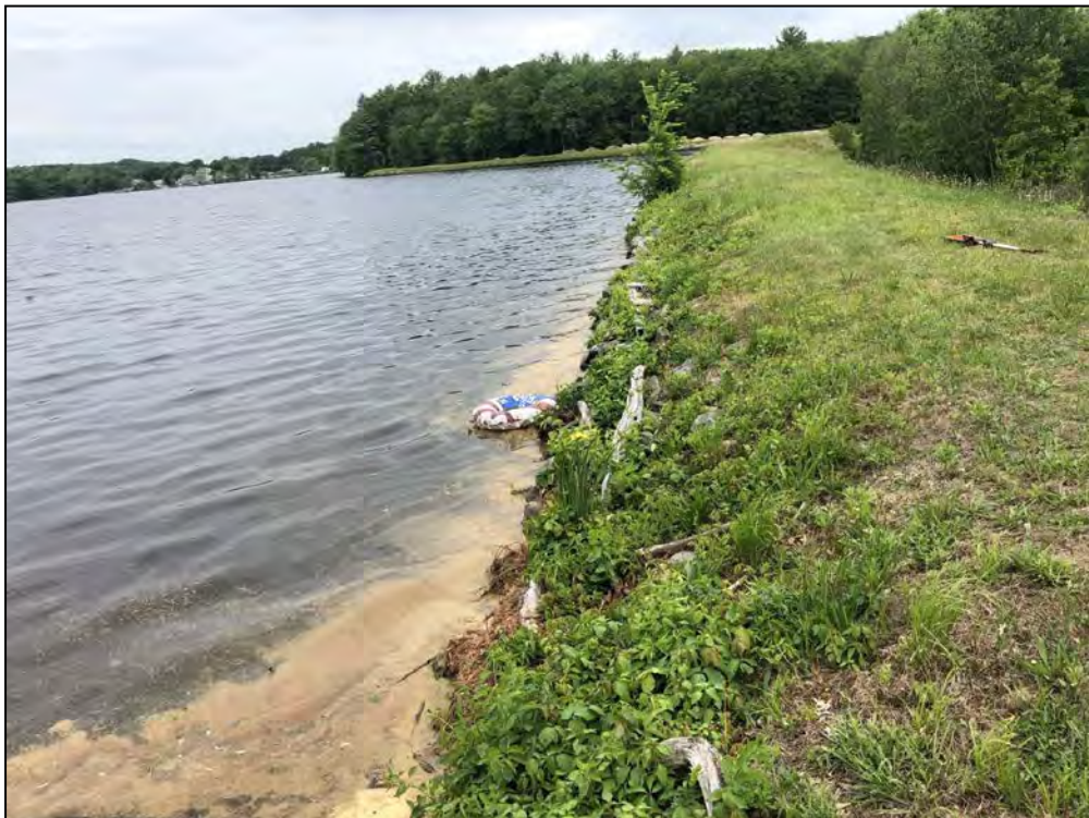
Photo No. 24: Bookers Dam - Upstream slope from near STA 3+00 looking left.
