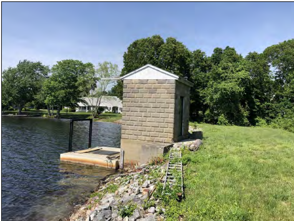
Photo No. 14: Main Dam - Upstream end of the outlet structure.
