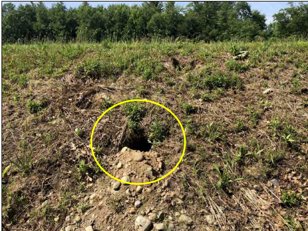
Photo No. 32: Bookers Dam - Typical active animal borrow near 4+00 along the downstream side of the embankment. Note the fresh gravelly-sand spoils along the underside of the borrow.
