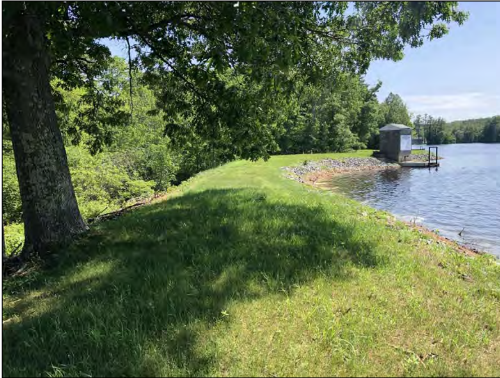
Photo No. 5: Main Dam - Crest from left abutment looking right.
