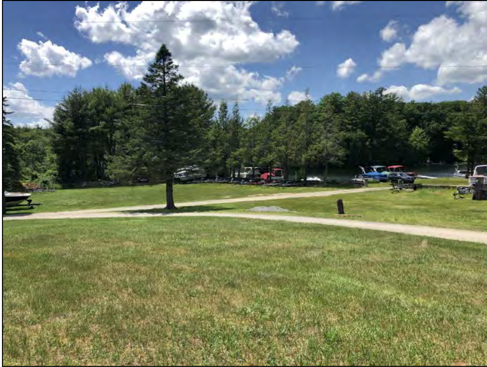
Photo No. 43: Marina Dam – Downstream area of the marina dam
