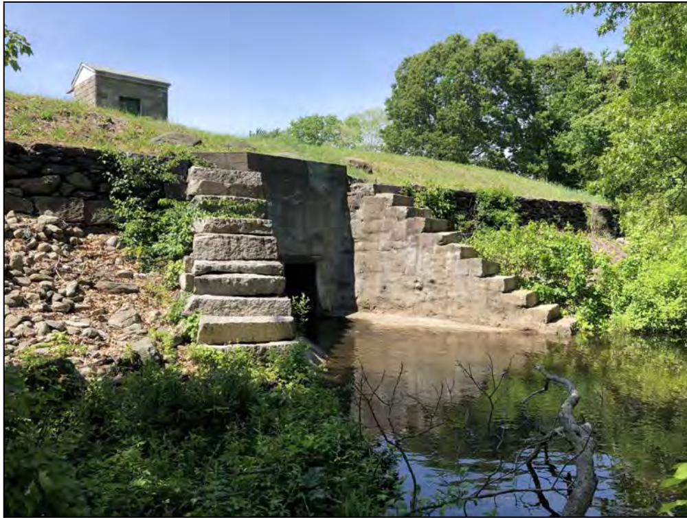
Photo No. 19: Main Dam - Overview of the discharge end of the conduit and the outlet left downstream channel wall.
