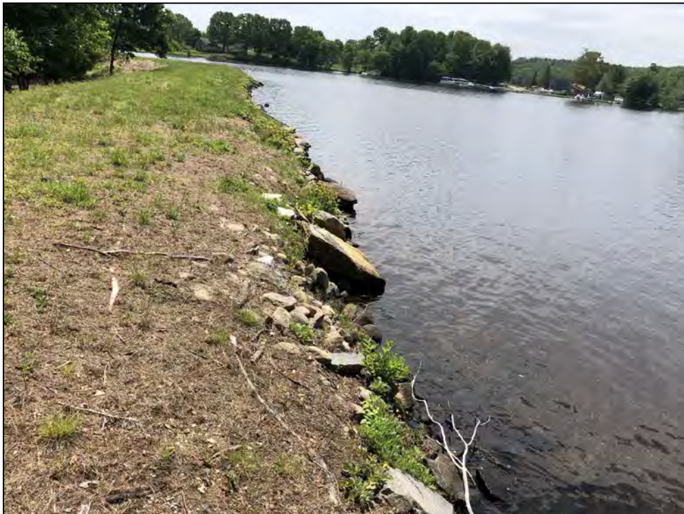
Photo No. 26: Bookers Dam - Upstream slope from near the right abutment looking right. Note the irregular alignment of the slope.
