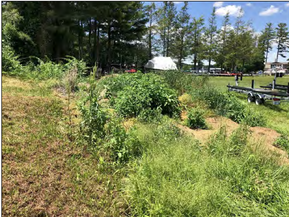
Photo No. 46: Pine Ledge Road to West Greenville Road Dam – Accumulated clippings and vegetation along the toe of the embankment left of Pine Ledge Road near the left abutment.
