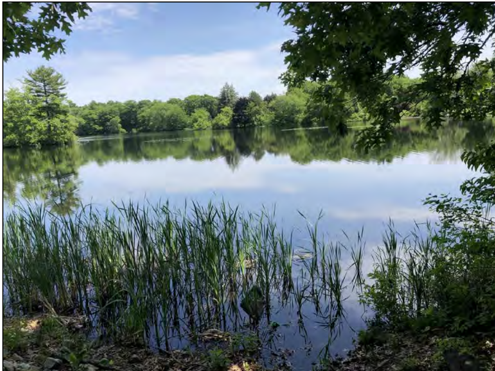
Photo No. 66: Spillway Section – Overview of the impoundment from the left abutment.
