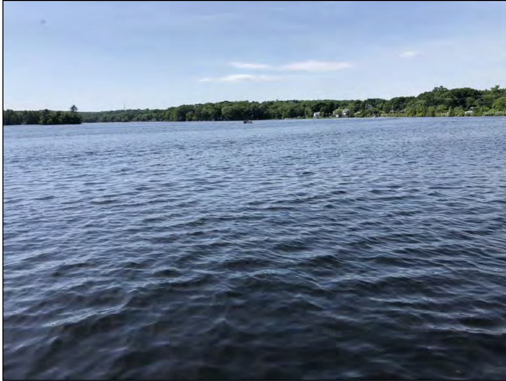
Photo No. 21: Main Dam - Overview of the impoundment.
