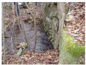
Seepage/leakage at Blue Dam (No. 229), Hopkinton
