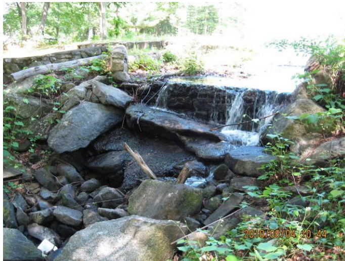
Spillway at Oak Swamp Dam (No. 168), Johnston
