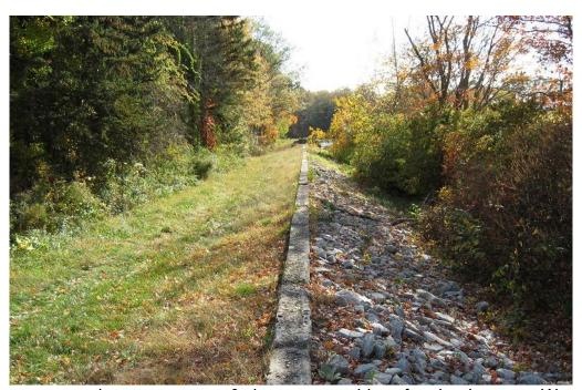
Improper vegetation on upstream & downstream sides of embankment at Waterman Dam (No. 111) in Glocester/Smithfield
