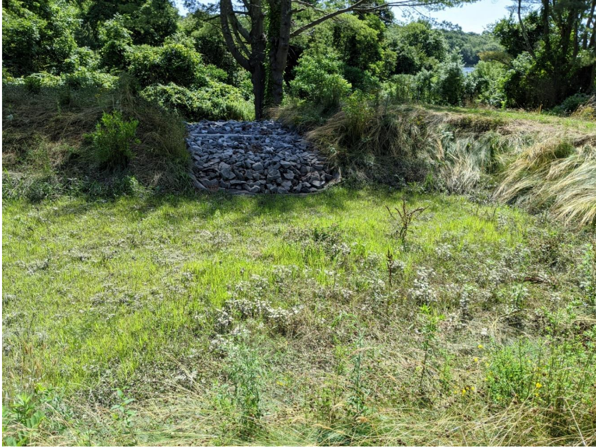
North Pond Stormwater BMP
