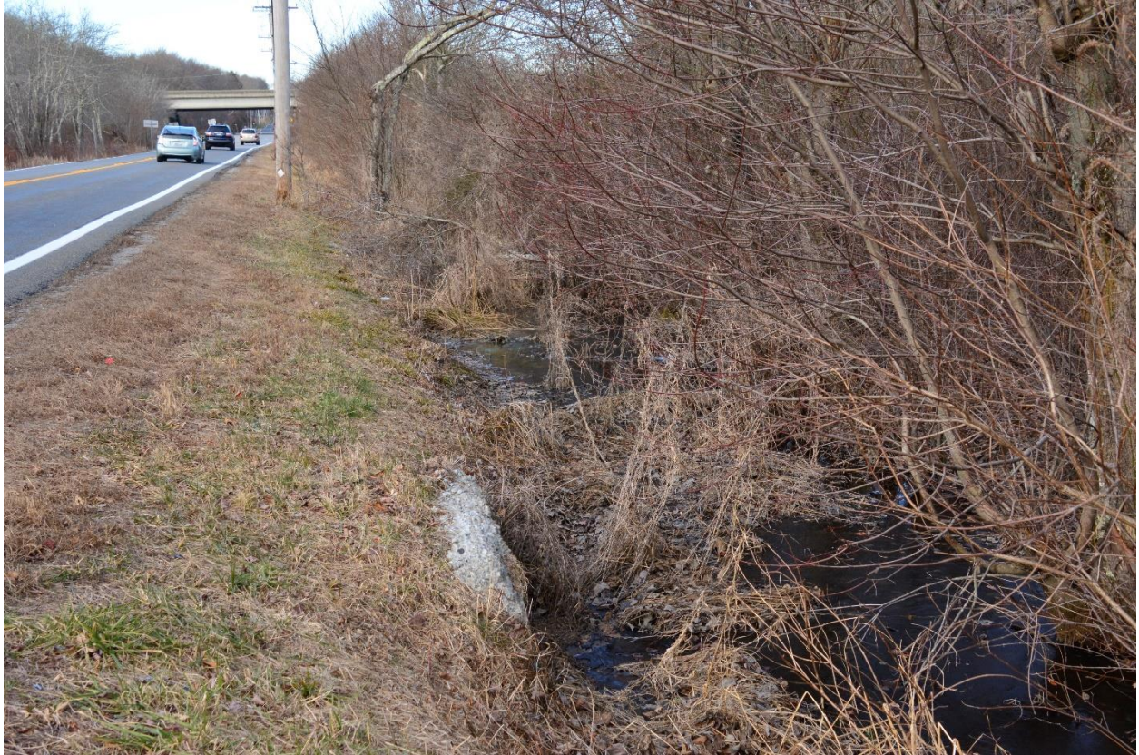
North Road crossing Jamestown Brook
