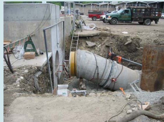
West Warwick WWTF Upgrade
