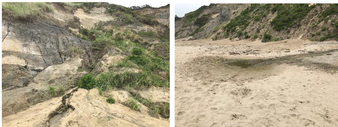
Figure 15: Sources 14W-1302 (left) and 14W-1319 (right) are both groundwater seeps flowing down the bluffs to the west of the Mohegan Bluffs trail head parking area
