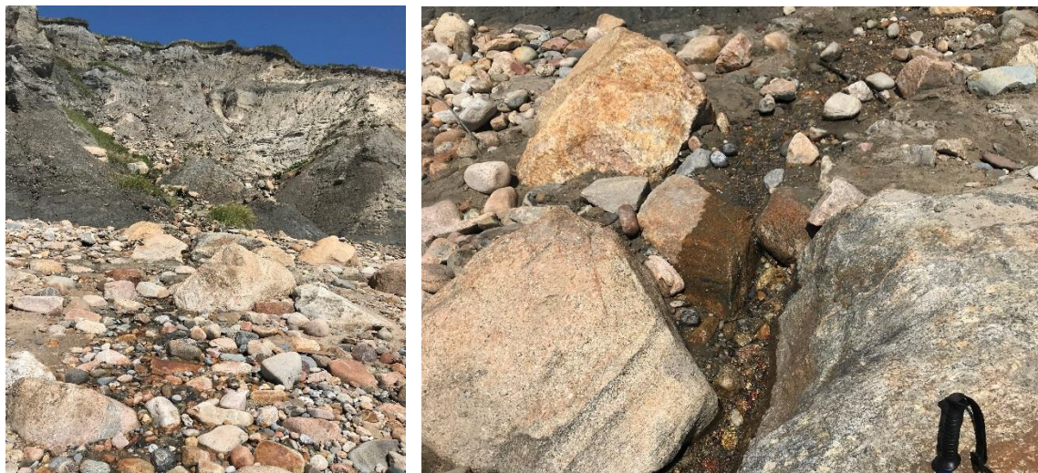
Figure 16: Sources 14W-1301 (left) and 14W-1328 (right) are groundwater seeps flowing down the bluffs to the east of the Mohegan Bluffs trail head parking area.
