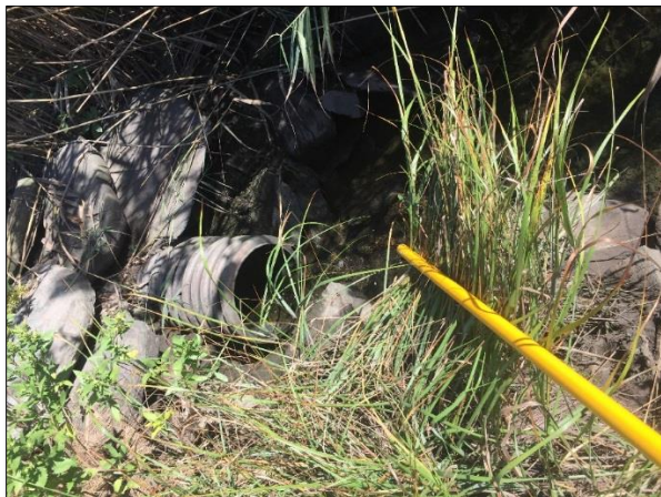
Figure 5: Source 7-803, a corrugated metal pipe discharging into the prohibited waters of Sheffield Cove in Jamestown, RI.
