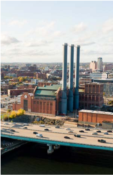
Manchester Street Power Station, Providence
