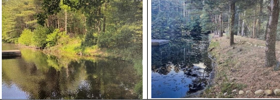
Wright T. Farm Dam (No. 587), Gloucester, View of upstream embankment before and after removal of excess vegetation-Pare 2021 inspection and 2022 inspection.
