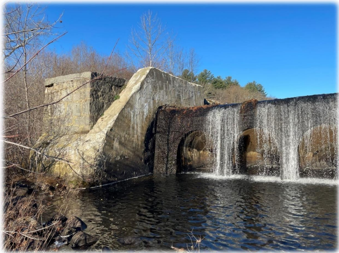
Hope Dam (No. 160), Scituate
