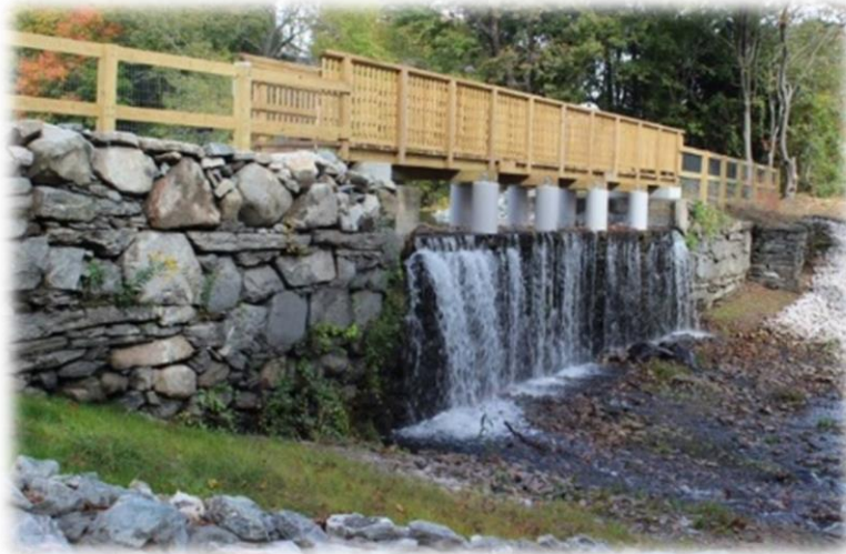
Silver Spring Dam (No 444). Photo dated October 18, 2022
