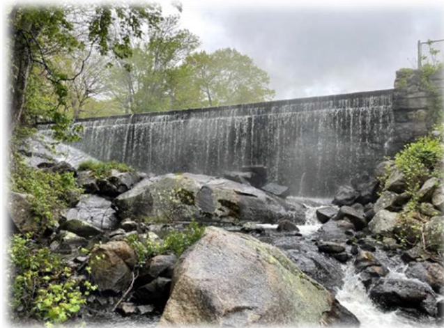
Boone Lake (No. 219) Downstream face of spillway – Pare Inspection May 19, 2022
