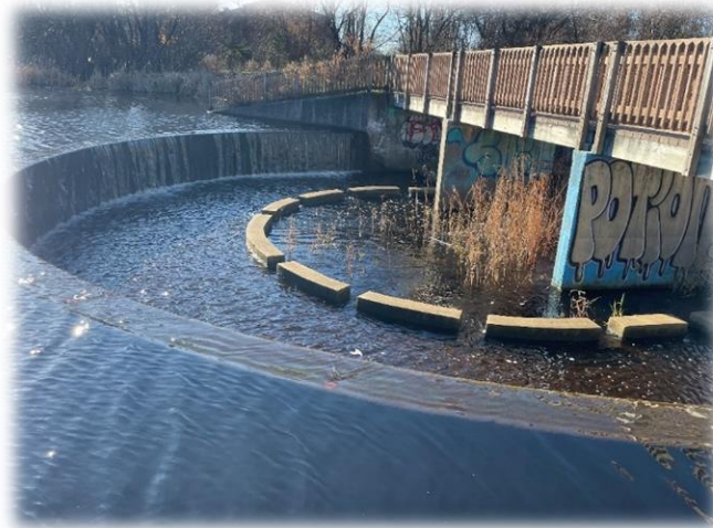
Indian Run Dam (No. 573), Spillway – RIDEM Inspection December 2022
