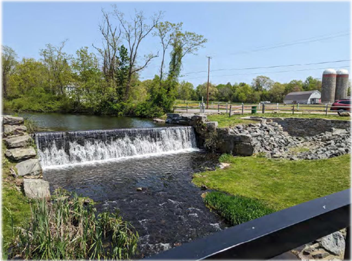
Butterfly Pond Dam (No. 097), Lincoln Photo taken by PARE Inspection - May 11, 2023
