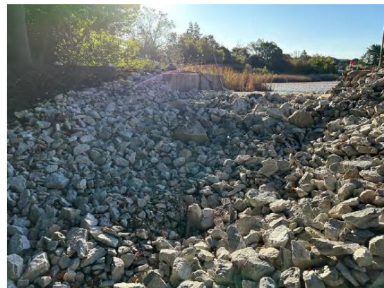
Stone Pond Dam (No. 320 ), Cranston, View of downstream auxiliary spillway before and after of fixing the spillway- GZA 2022 inspection and 2023 inspection.
