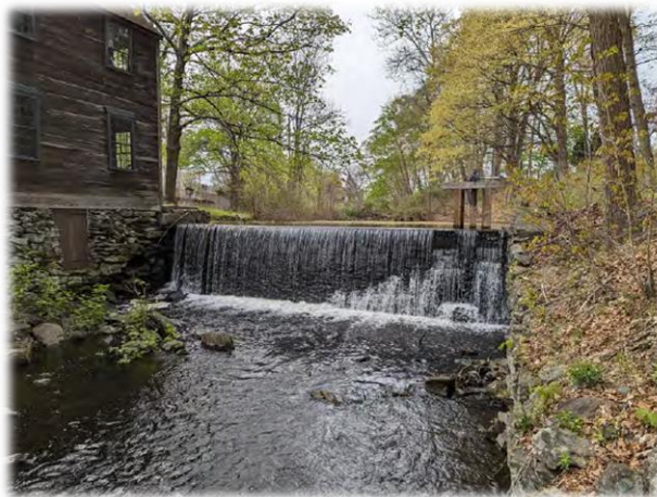
Moffett Dam (No. 099) Pare Inspection April 28, 2023
