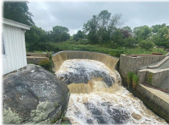
Horseshoe Falls Dam (No. 573), Primary spillway – GZA Inspection June 28, 2023
