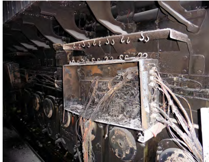
Figure 39: Fire damage to containership Gunde Maersk 's auxiliary engine no. 1 inboard side, looking forward.
