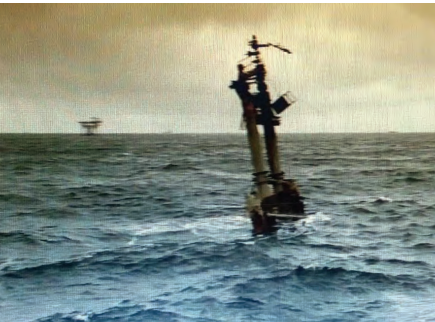
Figure 2: South Timbalier 271A platform after the allision and fire.
