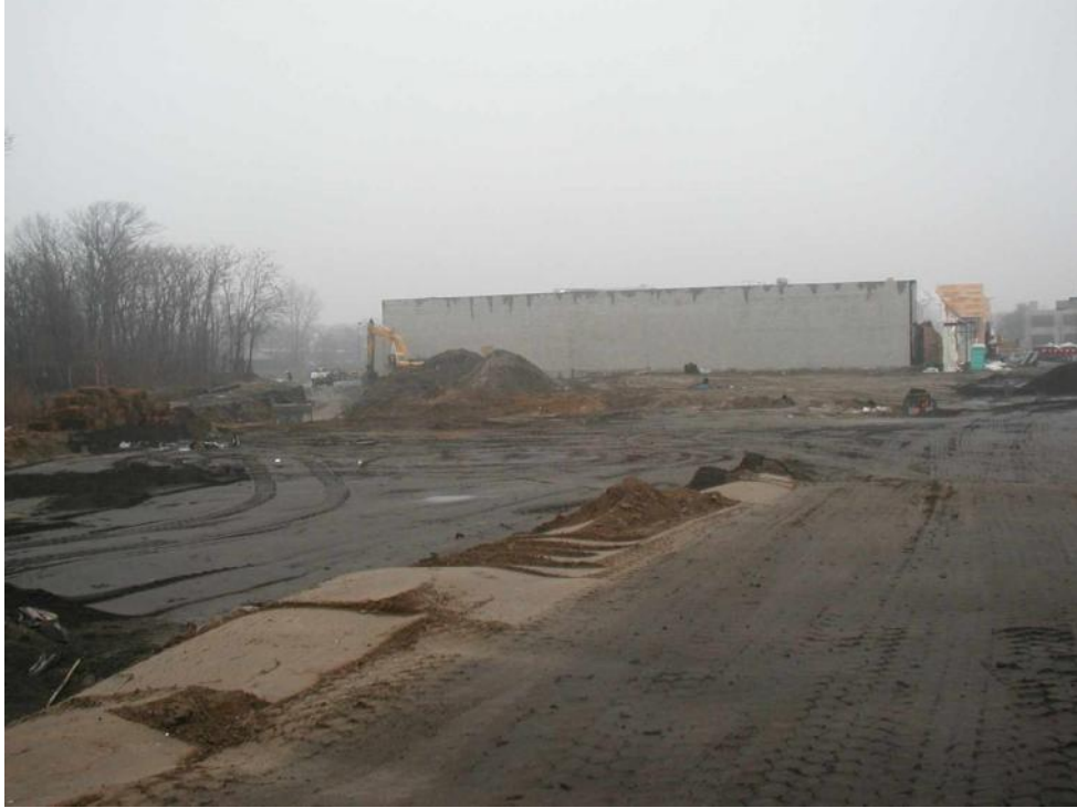
Photo 17. View east from southwest corner of excavation with backfilling nearly complete.
