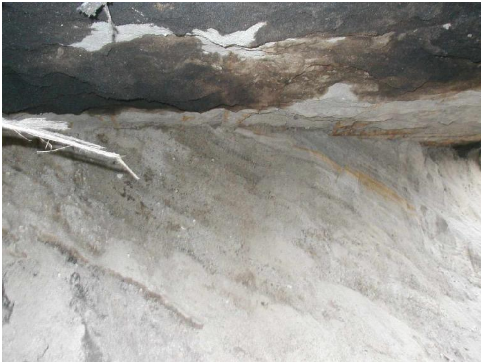
Photo 12. Clean soils directly beneath bunker.
