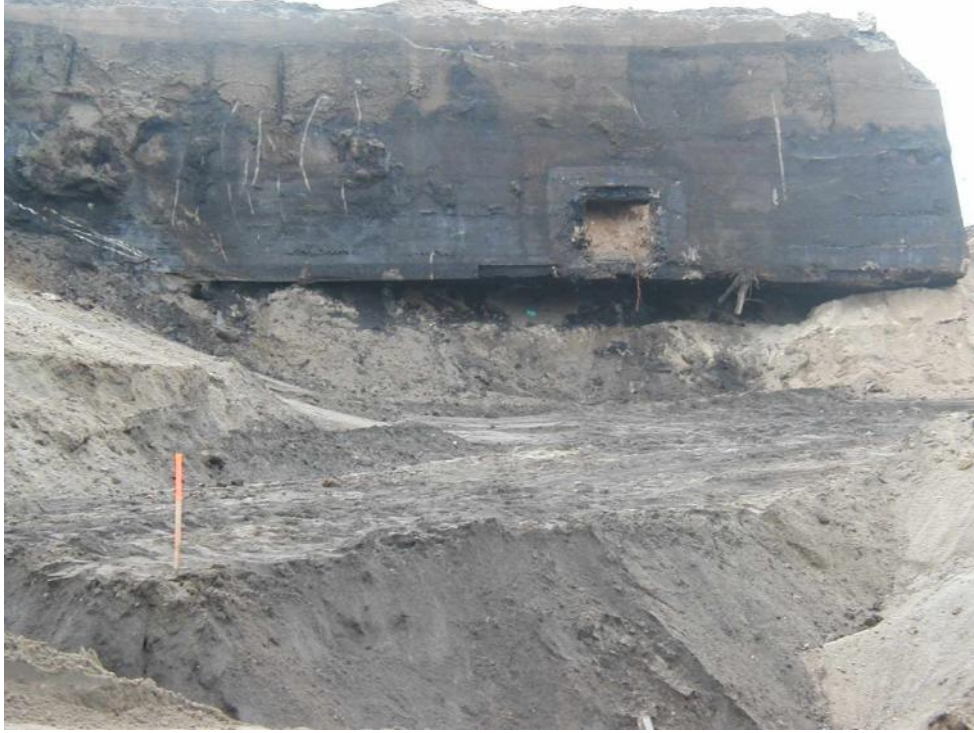
Photo 7. View west towards concrete bunker prior to removal of foreground soils.
