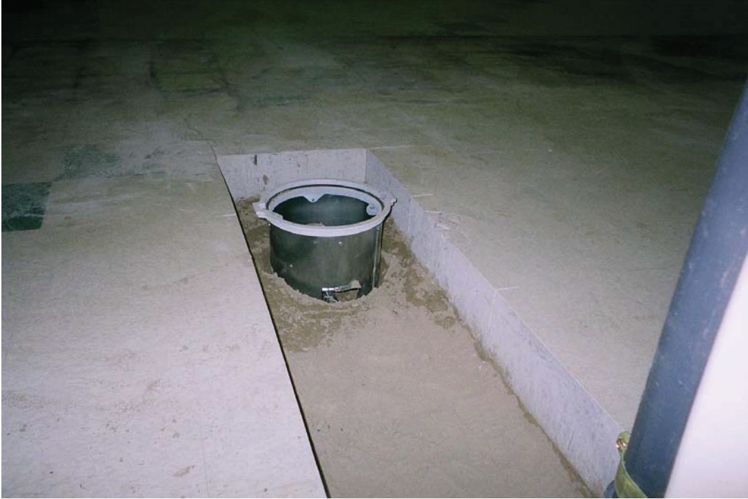
Extraction Well Vault Pre-pour
