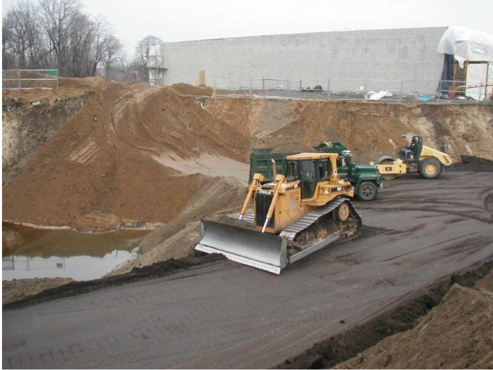
Photo 5. Backfill and compaction at east end of NAPL excavation.
