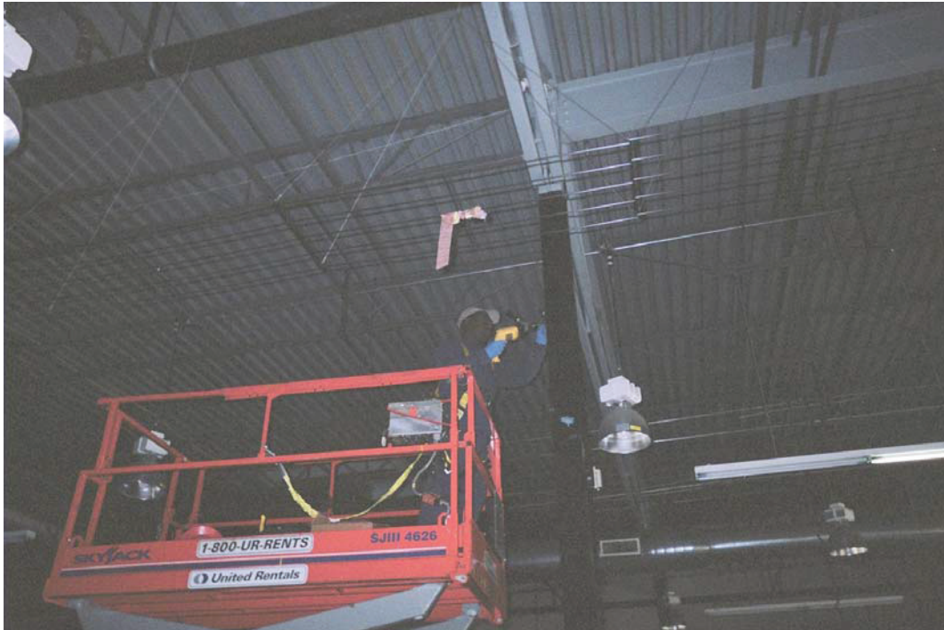
EW-7 Installation on Column
