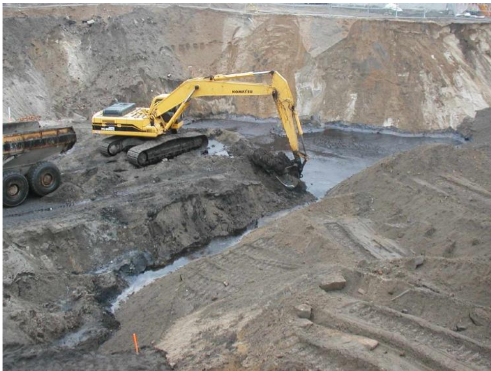
Photo 2. Removing NAPL soils.
