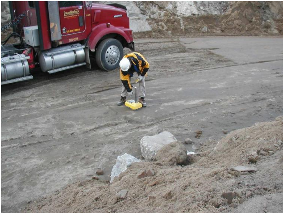
Photo 6. Compaction testing with nuclear density gauge.
