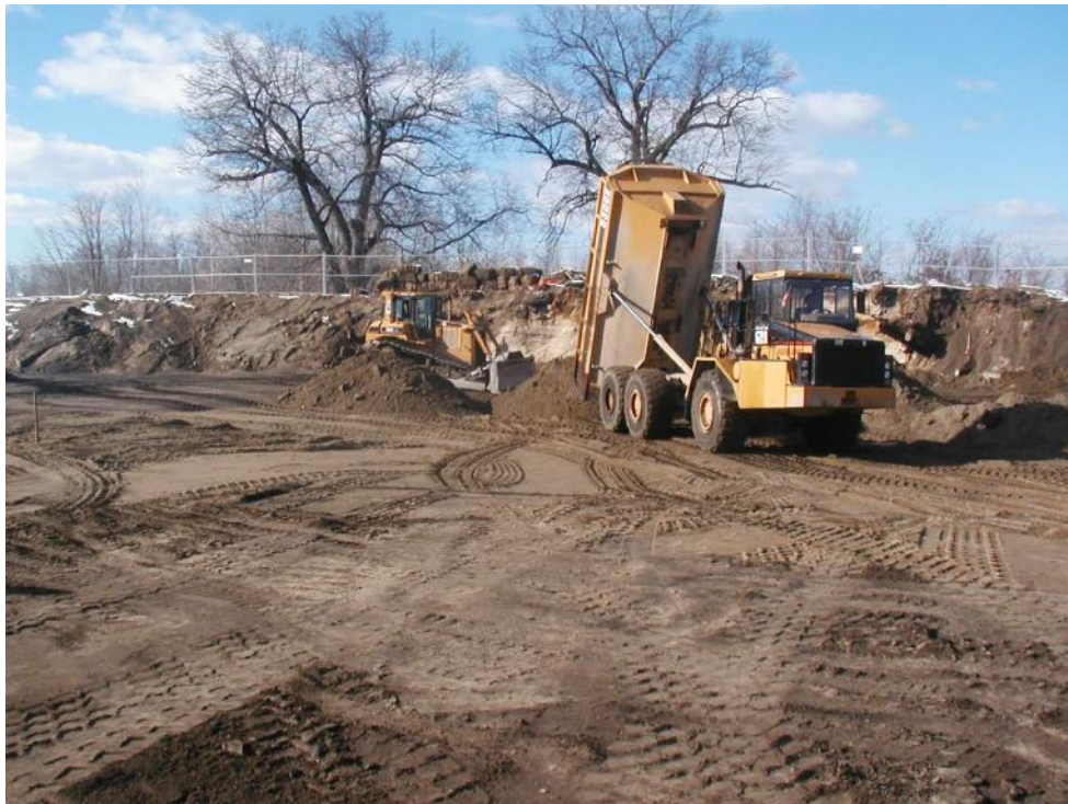
Photo 14. View northwest during backfilling.
