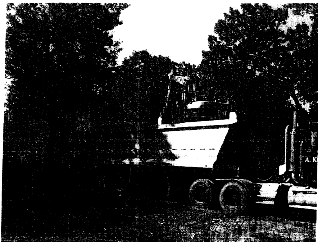
Progress Photo of Removal Activities in Main Soil/Debris Area
