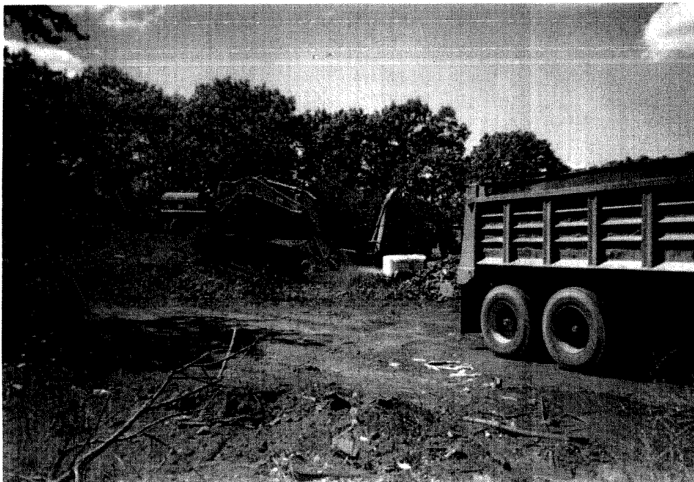
Soil/Debris Removal and Dust Suppression Activities in Main Soil/Debris Area
